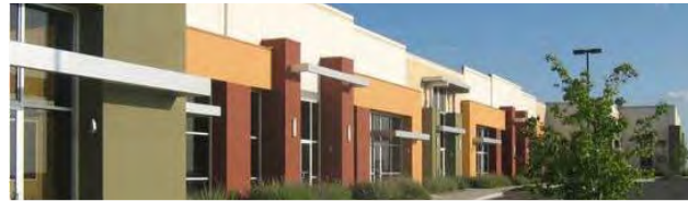
Articulation and color changes help to visually break up a much larger building into smaller pieces
