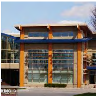
Entrance is celebrated with additional windows and unique architectural features
