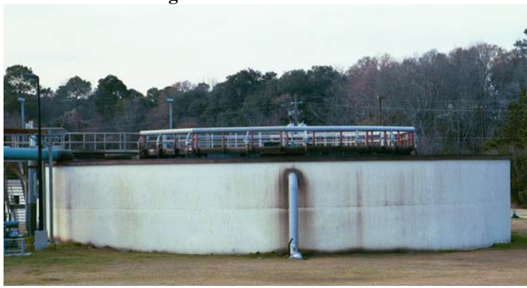
Figure 4.5 Package Plant - Point Peter WWTF
