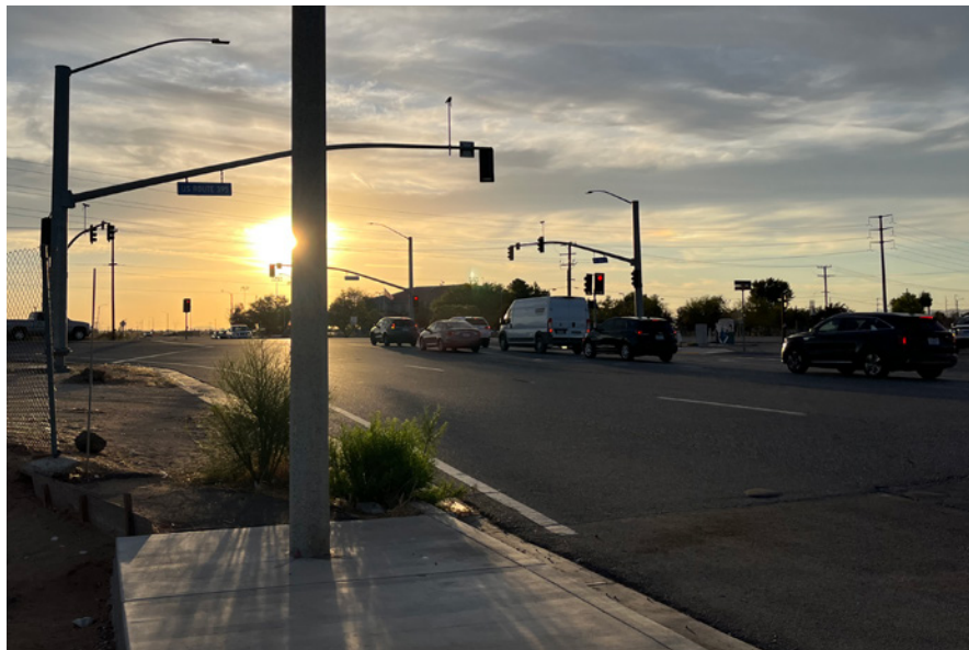
Sidewalk gaps along Air Expressway Boulevard were a common theme raised by community members during a pop-up event at Adelanto City Hall.
