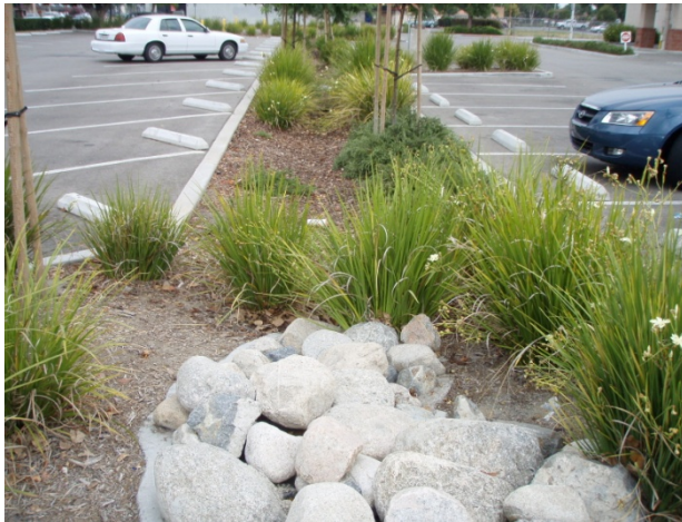
Parking lot vegetated swales collect rainwater and filter out toxic pollutants such as oils
