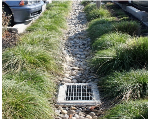
Bioswales in parking lots help filter out pollutants
