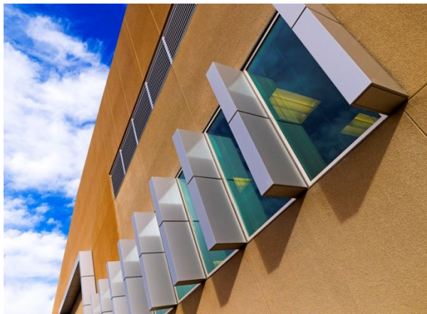
Window shades and awnings along south-facing building façade help block direct sun light and keep building interiors cooler, while allowing indirect natural sun light to illuminate interior spaces
