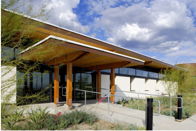
Overhangs reduce direct sunlight during the summer
