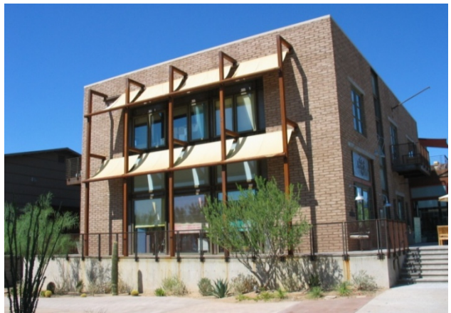
Window shades and awnings along south-facing building façade help block direct sun light and keep building interiors cooler, while allowing indirect natural sun light to illuminate interior spaces
