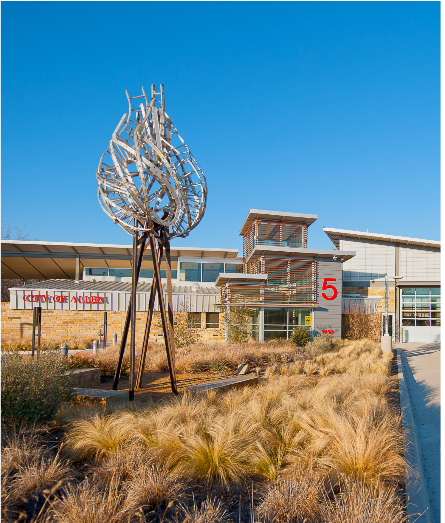
Christopher Fennell, Rail Ladder Fire , City of Allen Fire Station #5, 2011
