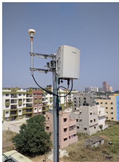
Example of Small Cell Wireless Facilities
