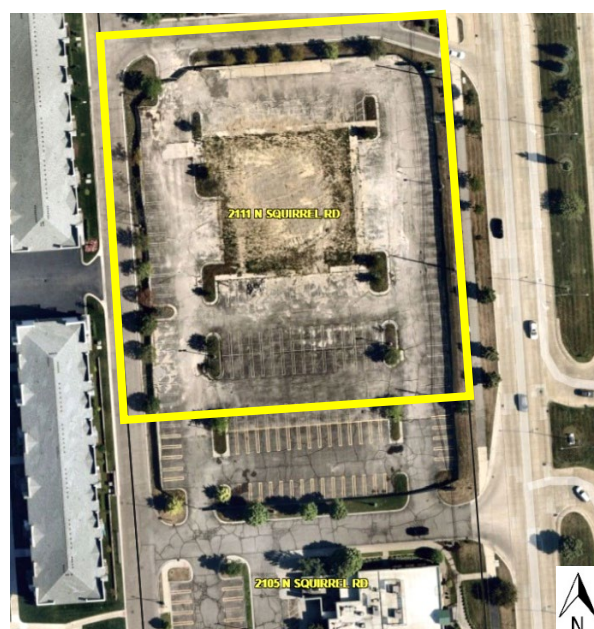
Building demolished – 2023 aerial photo
