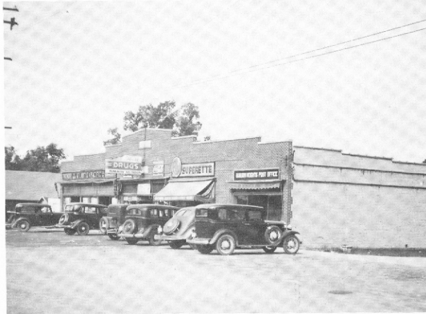
North side of Auburn Road: Shearer block,
