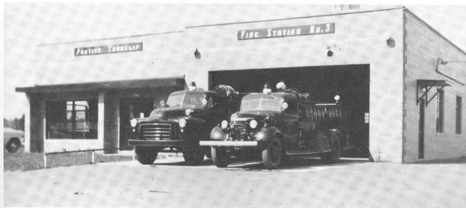
Fire Station No. 3, Joslyn Road
