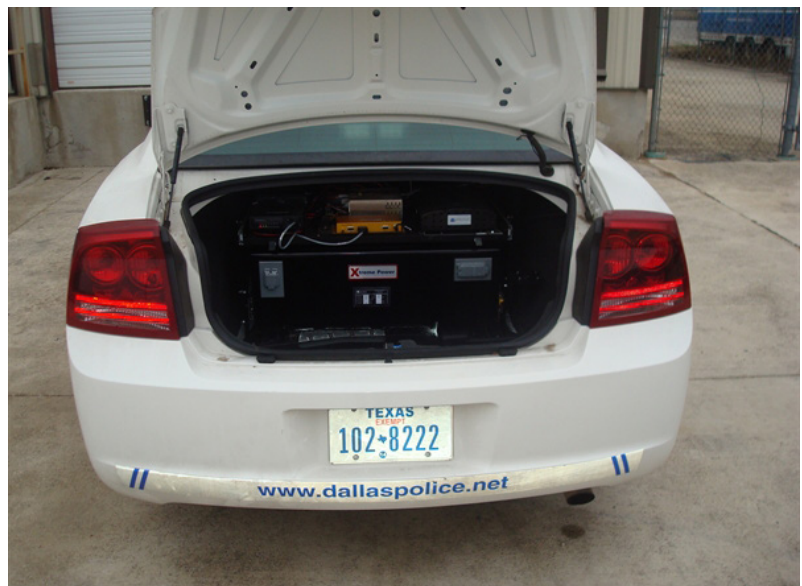
Figure 3: EnergyXtreme system installed in the trunk of a Dodge Charger owned by the Dallas, TX police department.
