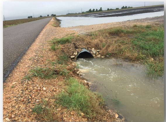
Side road pipe on Lindermann Rd.
