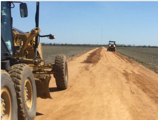
Construction crews work on Lindemann Rd.
