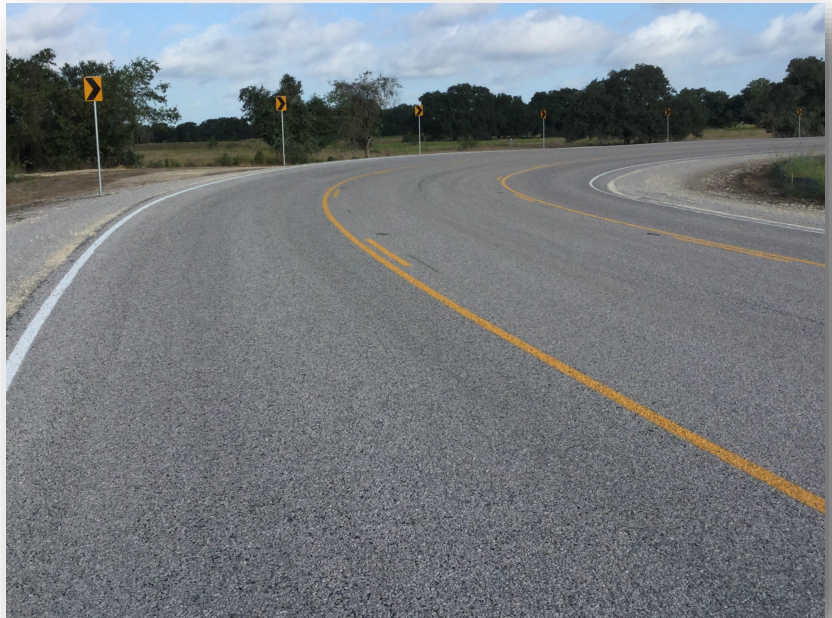
Striping on Williams Rd. (Pct. 2)
