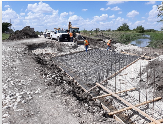
Bridge crew at Stockton culvert site.
