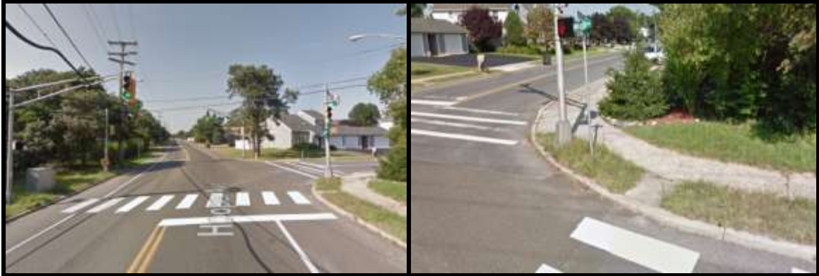
Figure 36: Improved pedestrian crosswalks and lights at intersection of A Street & Hooper Avenue, Seaview Village; however, detail (right) shows non-ADA compliant ramps and sidewalks (Google Streetview)
