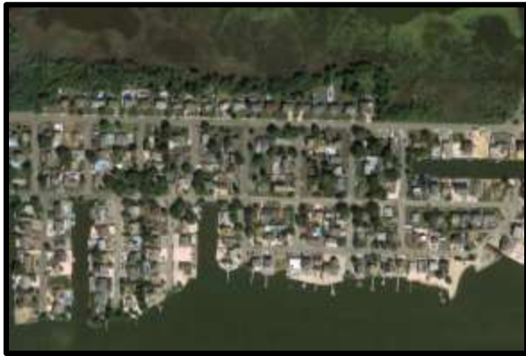
Figure 17: Aerial of eastern portion of Bay Harbor (Google Maps)
