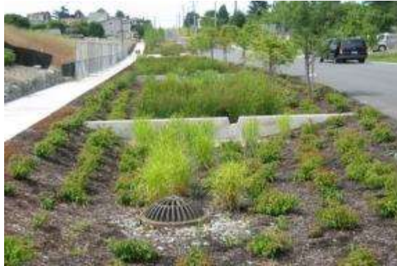
Figure 127: Example of a streetside bioswale ( www.kwalliance.org )
