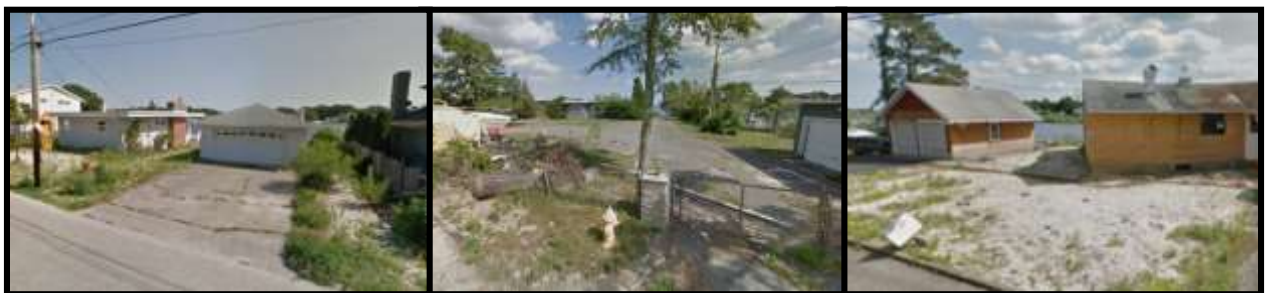
Figure 131: Examples of vacant or abandoned buildings in Cherry Quay-Bay Harbor (Google Streetview)
