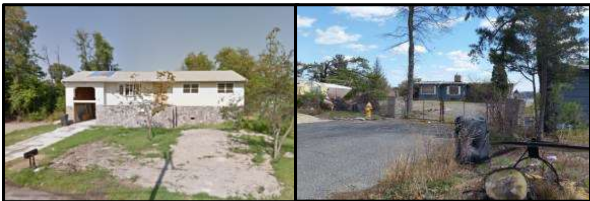
Figure 31: Damaged/Gutted homes (Google Streetview; Site visit – April 24, 2015)
