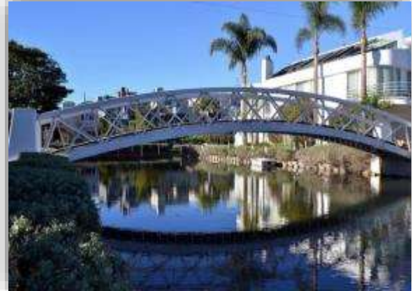
Figure 118: Example of a pedestrian bridge in a residential neighborhood (Credit: Amatullah Guyot http://www.welikela.com/top-10-los-angeles-bridges-to-photograph/ )
