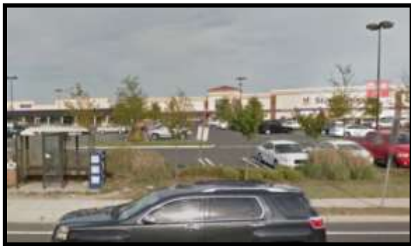
Figure 106: Front view of the shopping center on Brick Boulevard (Google Streetview)
