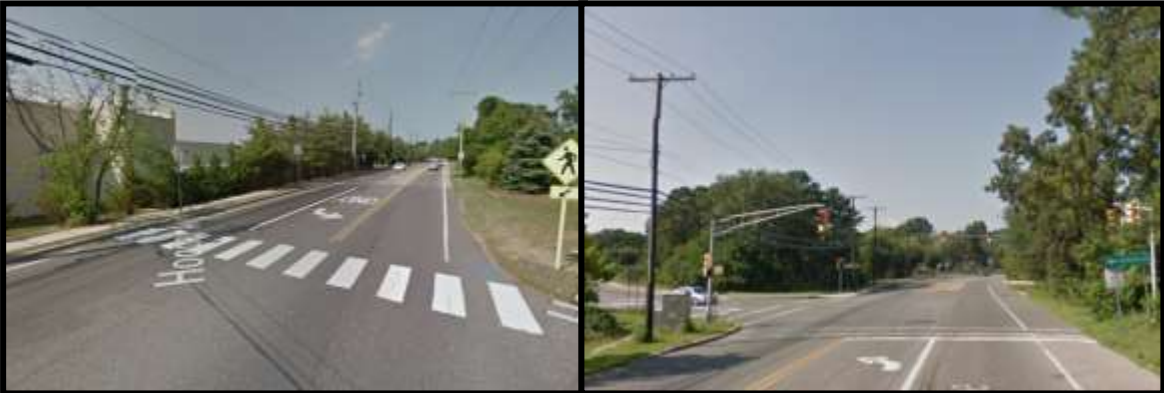
Figure 37: Left: A crosswalk on Hooper Ave. between Bay Harbor and back of shopping plaza with no sidewalk on one side and no ramp on the other; Right: Crosswalk without sidewalks at major intersection, Hooper Ave. & Beaverson Blvd. (Google Streetview)
