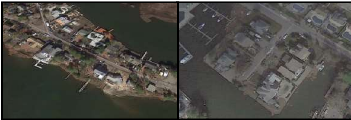
Figure 32: Storm damage in Mallard Point (average year built: 1970) versus Sailor's Quay (average year built: 1992) (Google Earth, Nov. 3, 2012)
