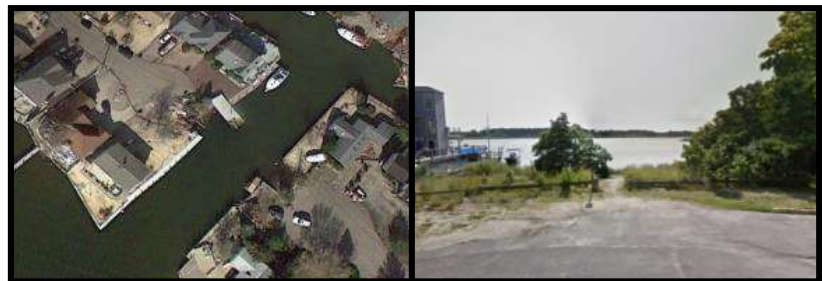
Figure 135: Images of street-ends in Cherry Quay that experienced heavy damage to bulkheads (left) and with right-of-ways/public access with natural shoreline (right) (Google Streetview)
