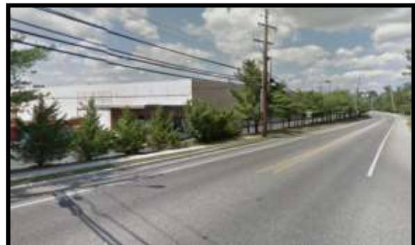
Figure 105: Rear view of the shopping center, Hooper Avenue (Google Streetview)
