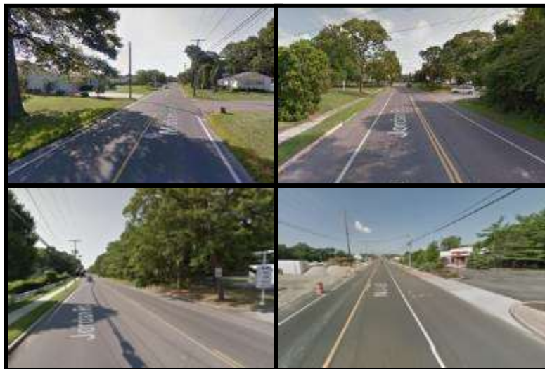
Figure 197: Examples of primary and secondary roads that could benefit from bicycle treatments (Google Streetview)
