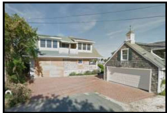
Figure 76: Damaged/Gutted home, Post-Sandy (Google Streetview)
