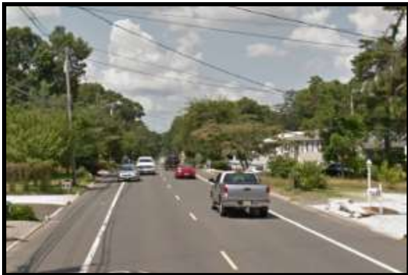
Figure 83: Busy road without sidewalks, Princeton Ave. (Google Streetview)
