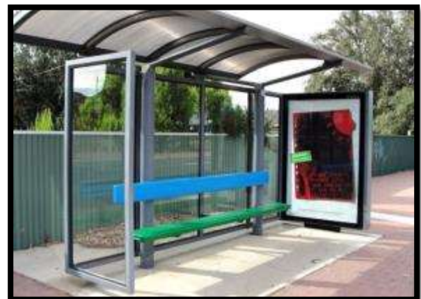
Figure 198: Example of a well-designed suburban bus shelter
