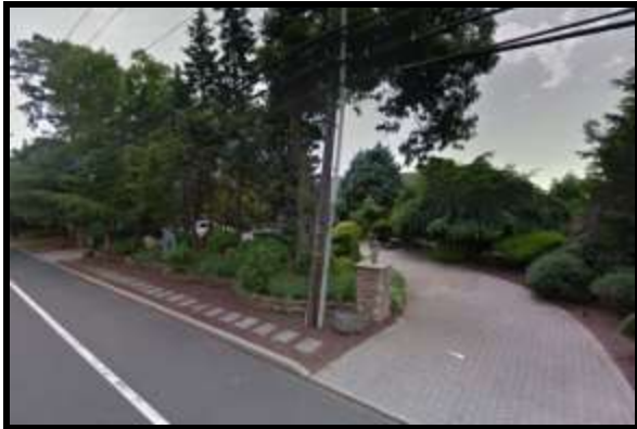
Figure 82: Decorative, but substandard sidewalk, Princeton Ave. (Google Streetview)
