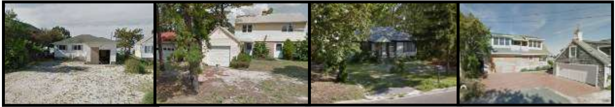
Figure 212: Examples of abandoned and/or unmaintained buildings throughout Princeton-Midstreams (Google Streetview)
