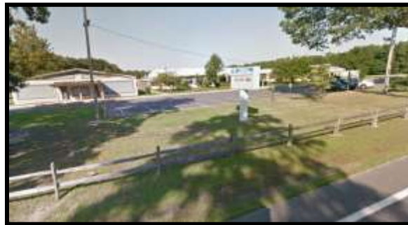
Figure 117: Front building façade and parking lot of Midstreams Elementary School (Google Streetview)
