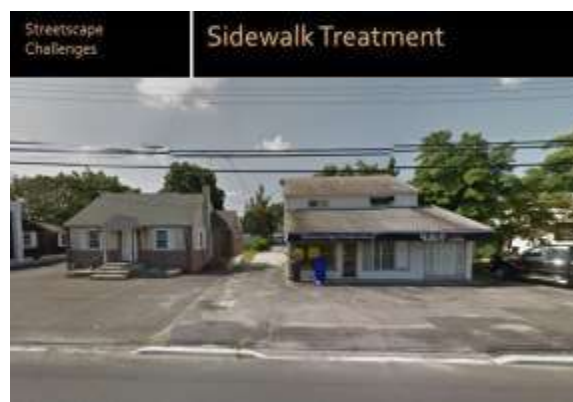
Figure 208: Sidewalks are missing in many areas of the neighborhood, particularly where lawns or parking take the place of the public right-of-way, such as this commercial area on Princeton Ave., Princeton (Google Streetview)
