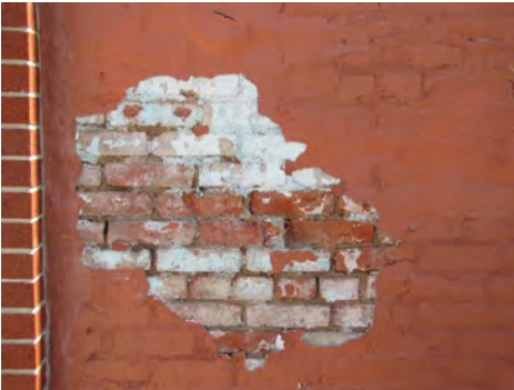
Above left: chipping paint on side façade. Above right: This siding hides the original materials of the building beneath and also creates a large, featureless expanse.
