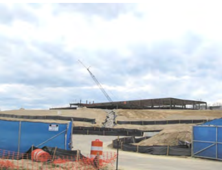
New construction near I-96 (Brighton, MI)
