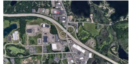
Grand River Avenue/I-96 Interchange
