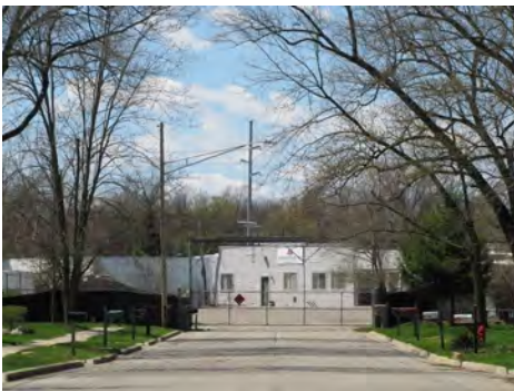
The images above show the variety of industrial areas in the city
