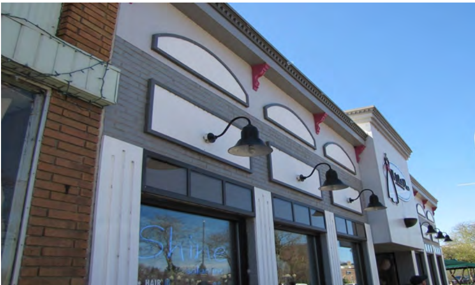
These gooseneck fixtures light the way for pedestrians passing beneath them and also function as a decorative element on the building façade.
