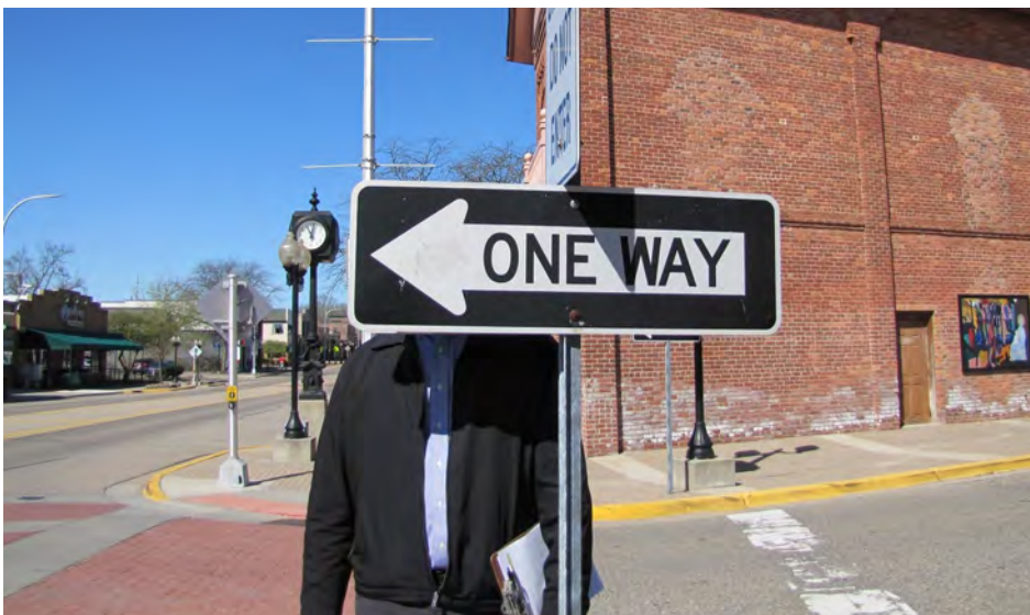
This is one example among many in the downtown of a uniform traffic control device that is installed with an inadequate clearance height.
