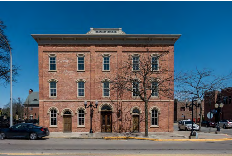
This former hotel has found new life as a modern brewery and restaurant; the new use preserves a piece of the city's history.
