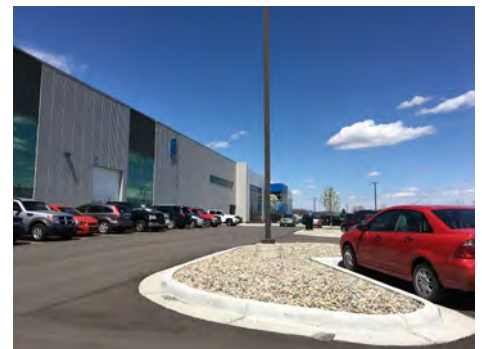
Industrial development located at the north end of the city.
