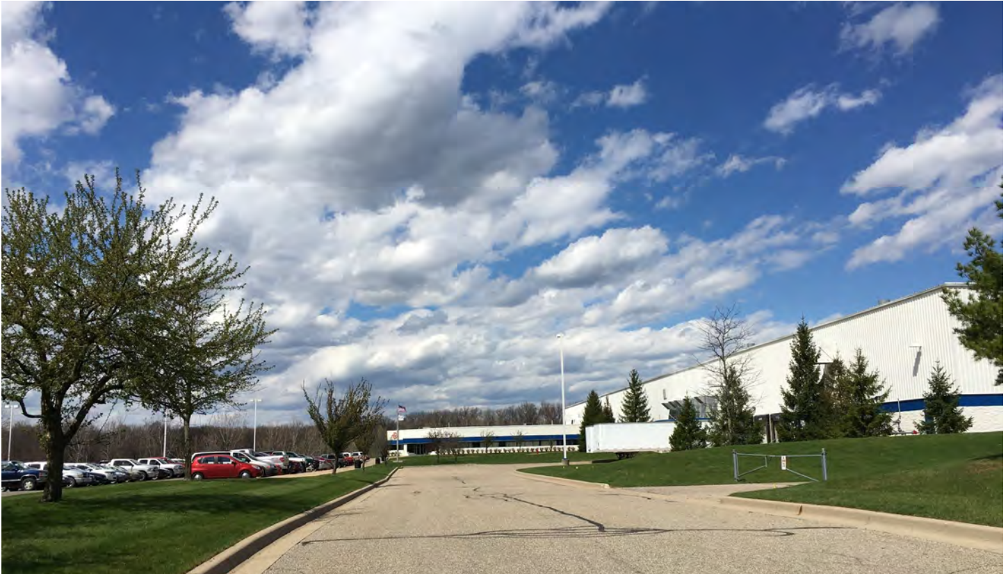
This industrial facility is located immediately west of the Challis Road redevelopment site. .
