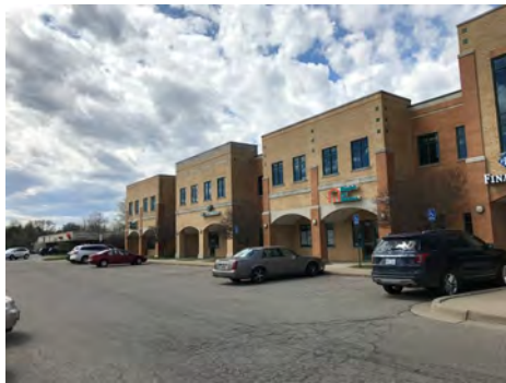
New construction on Grand River Avenue
