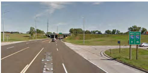
Grand River Avenue/I-96 Interchange
