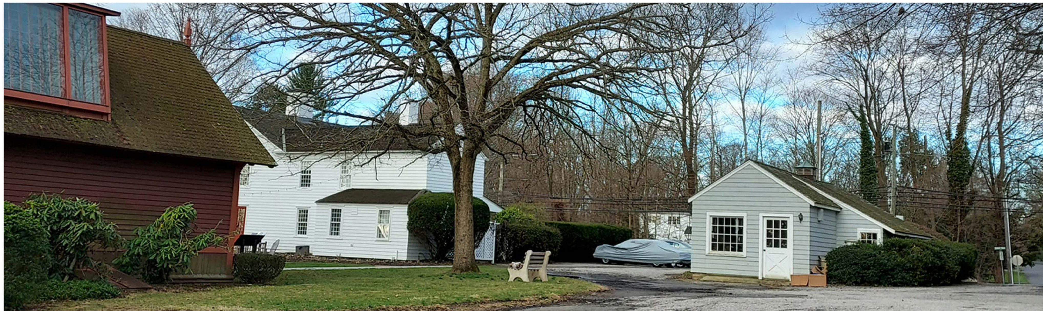
VIEW FROM PARKING - EXISTING
