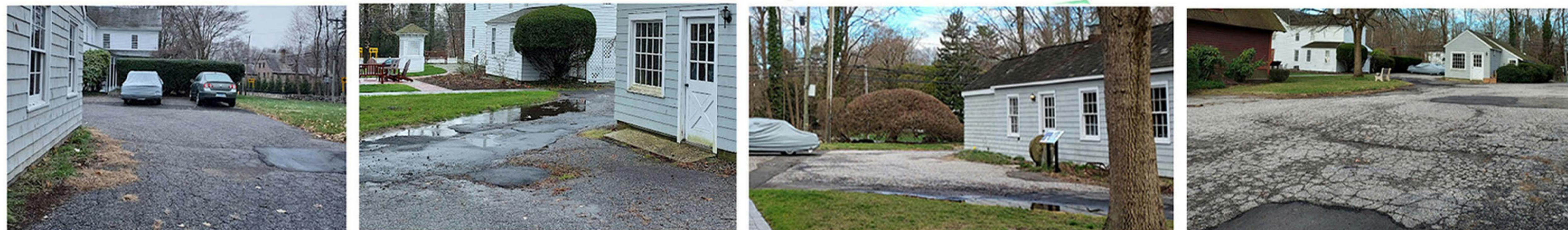
EXISTING PAVEMENT CONDITIONS
