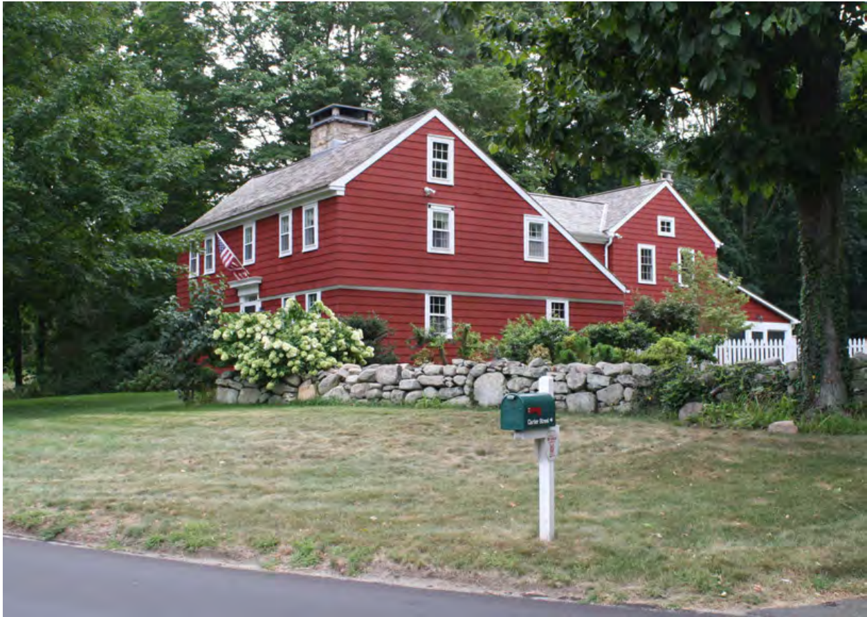
Figure 7. Northeast view of Benedict-Eels-Thatcher House; camera facing southwest.
