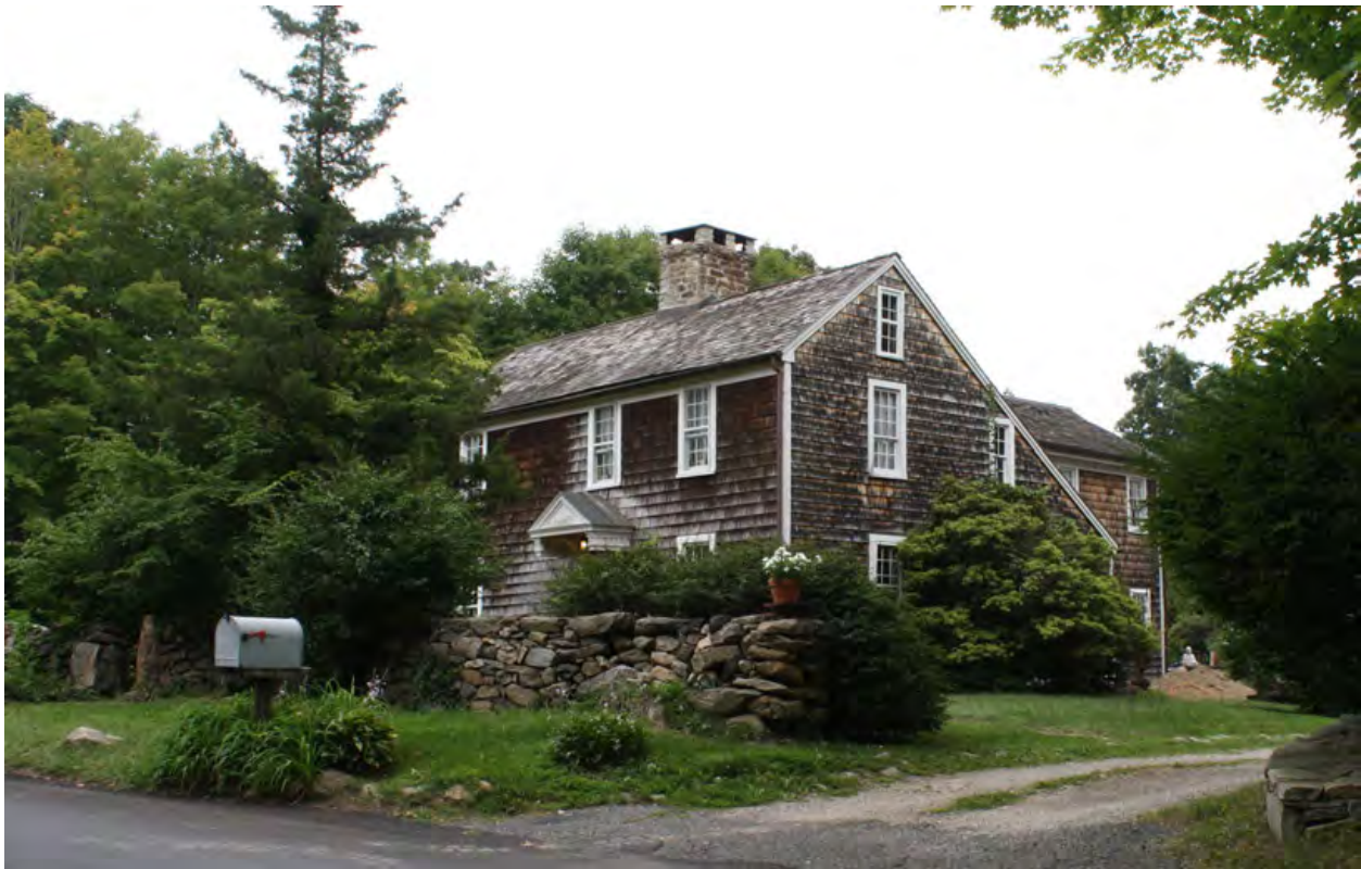
Figure 6. Southwest view of Fitch-St. John-Ruscoe House; camera facing northeast.
