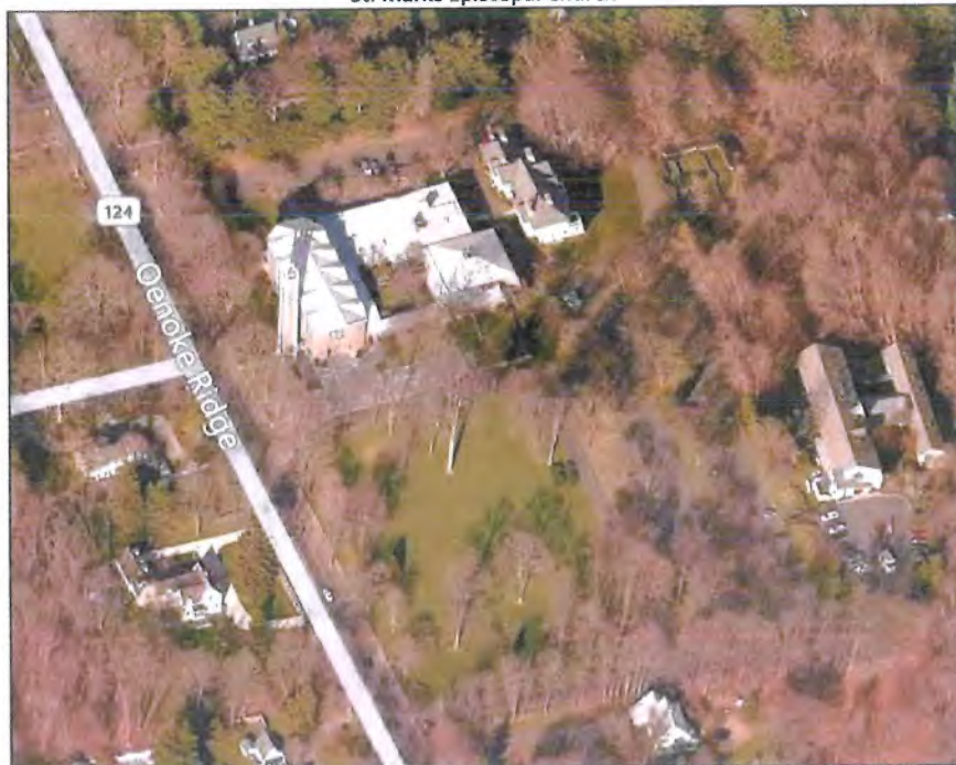
St. Marks Episcopal Church
