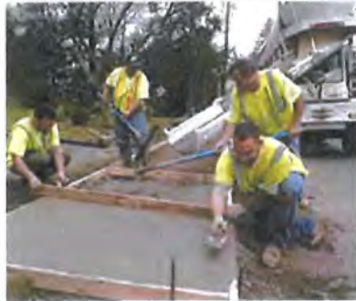
Main Street Sidewalk Construction
