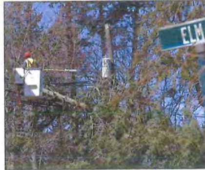
Electrical Service Interruption
