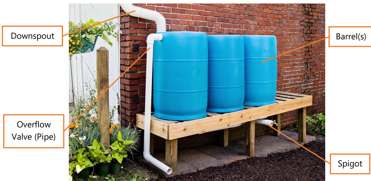
Figure 3. Rain barrels with labeled components.
