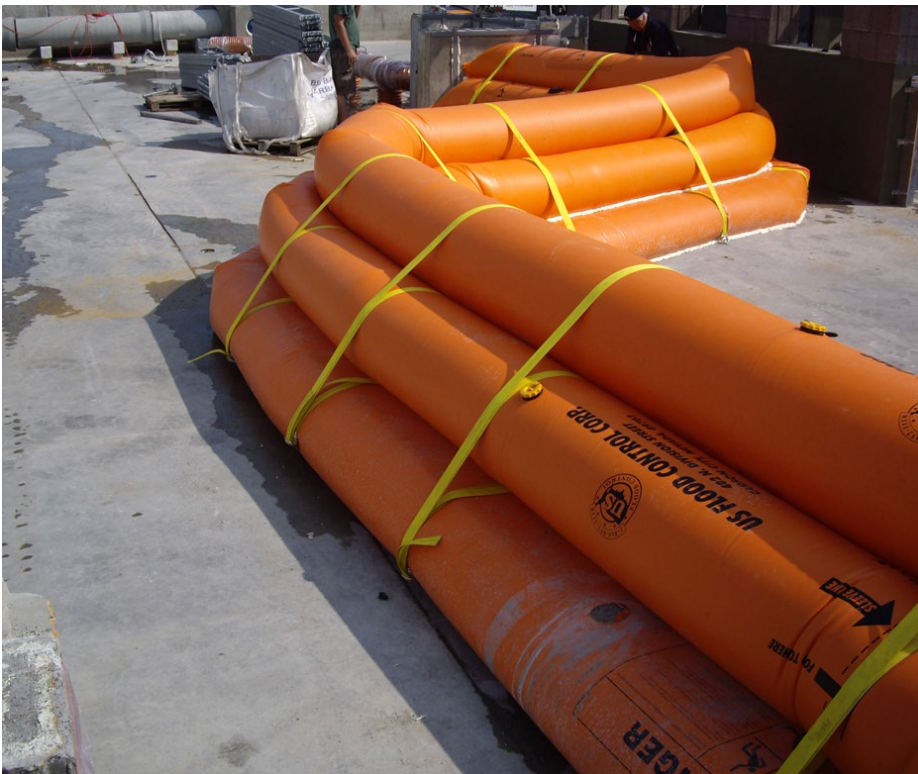
Figure 18. Example of a water inflated temporary dam system.
