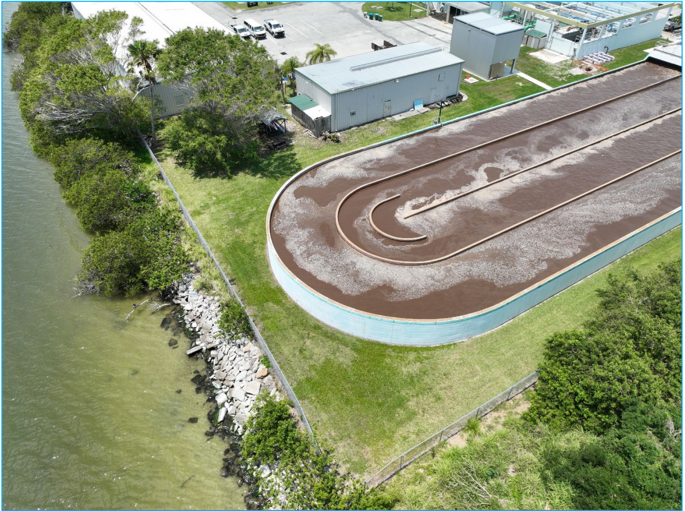
Figure 10. The WRF's Oxidation Ditch is located adjacent to the BRL.
