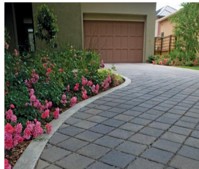
Pervious or Permeable Pavements
