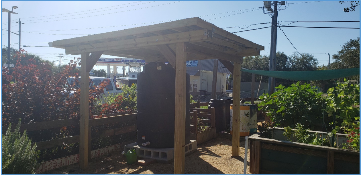
Figure 2. Cape Canaveral Community Garden. LID attributes include a 500-gallon rainwater collection tank and permeable coquina ground cover.
