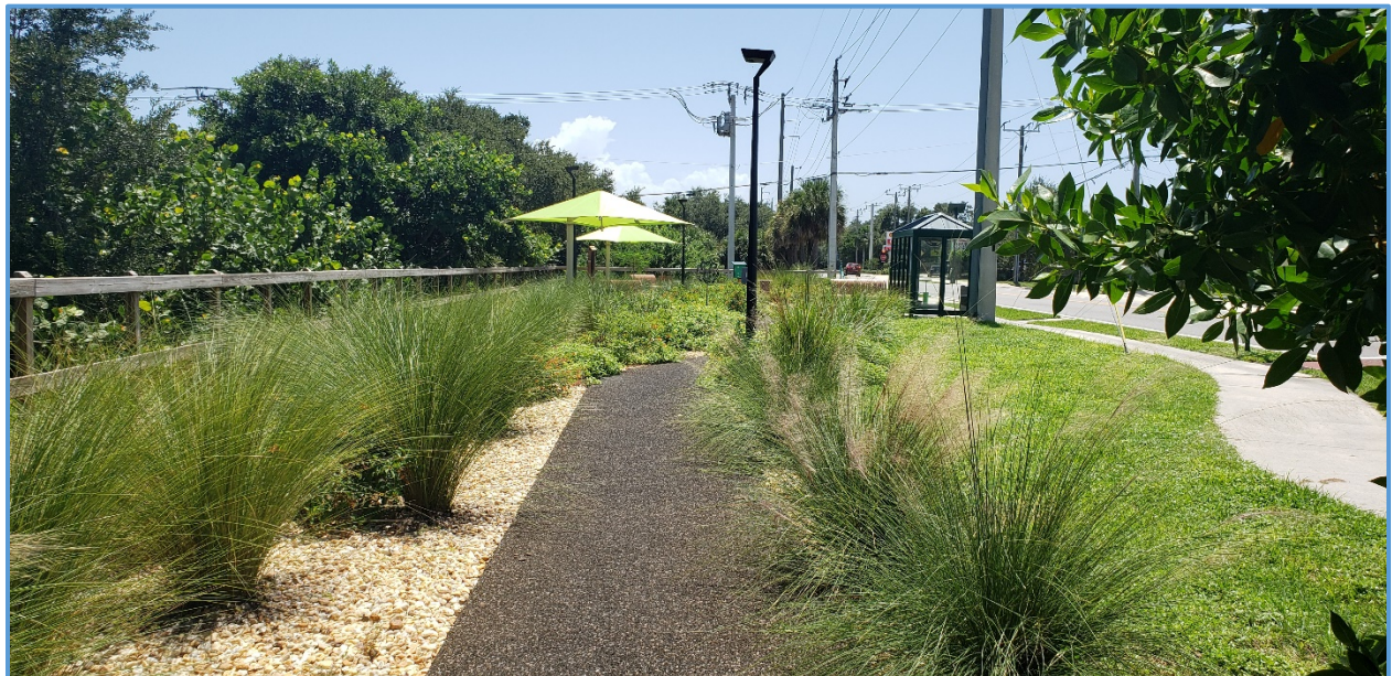
Figure 1. Wagner Park on North Atlantic Ave. LID attributes include permeable walkways, Florida native plants, a bioswale and limited use of grass as ground cover.
