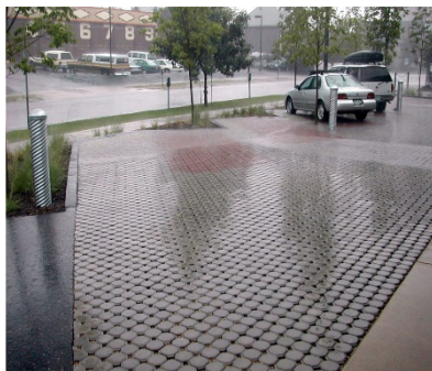
Pervious or Permeable Pavements
