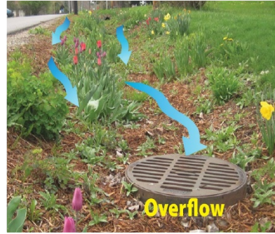
Overflow Channels or Drains
