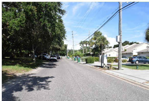
Overhead utilities along Washington Ave.
