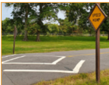
Speed Hump, Source: City of Winter Springs, FL
