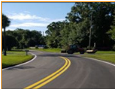
Repaved road in Pasco County, FL
