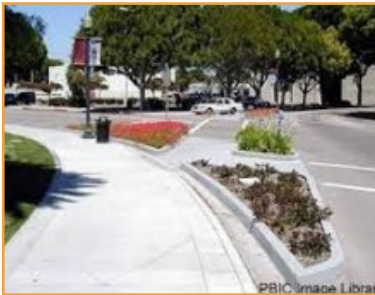
Reduced Curb Radius, Source: SRTS
