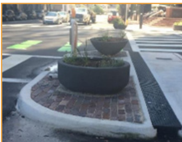
Curb Extension along SR 60/ Jackson Street in Tampa, FL
