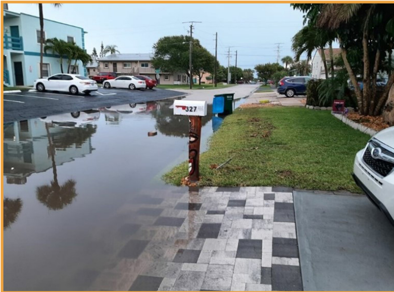
Localized flooding on Fillmore Ave
