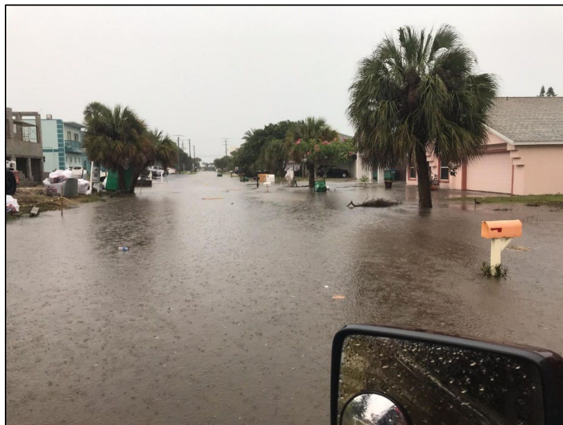
Storm-related flooding along Filmore Ave.
