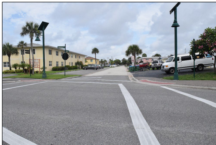
Pedestrian crosswalks at intersection of Monroe Ave. and Ridgewood Ave.
