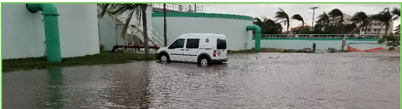
Figure 3. Flooding at the City’s Water Reclamation Facility after Hurricane Irma in 2017 due to a lift station backup.
