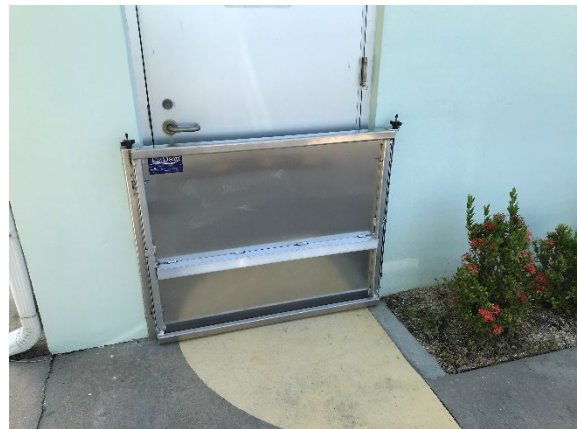
Figure 4. Semi-permanent flood barrier installed at the City's Water Reclamation Facility.
