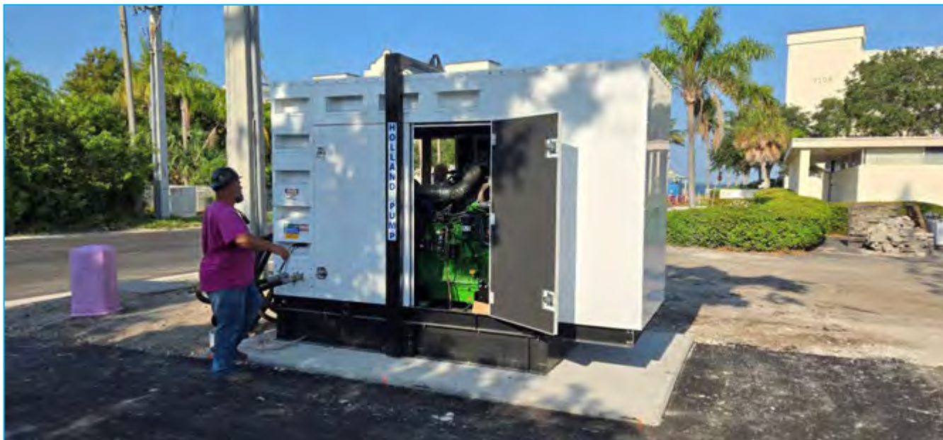
Figure 13. Center Street Pump Station.
