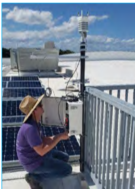
Figure 7. C5 weather station being installed by an FAU student.
