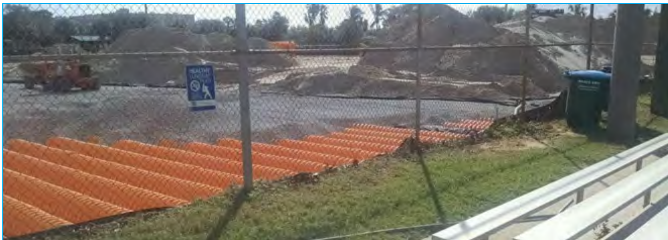
Figure 16. Stormwater exfiltration system under construction at Canaveral City Park in 2016.
