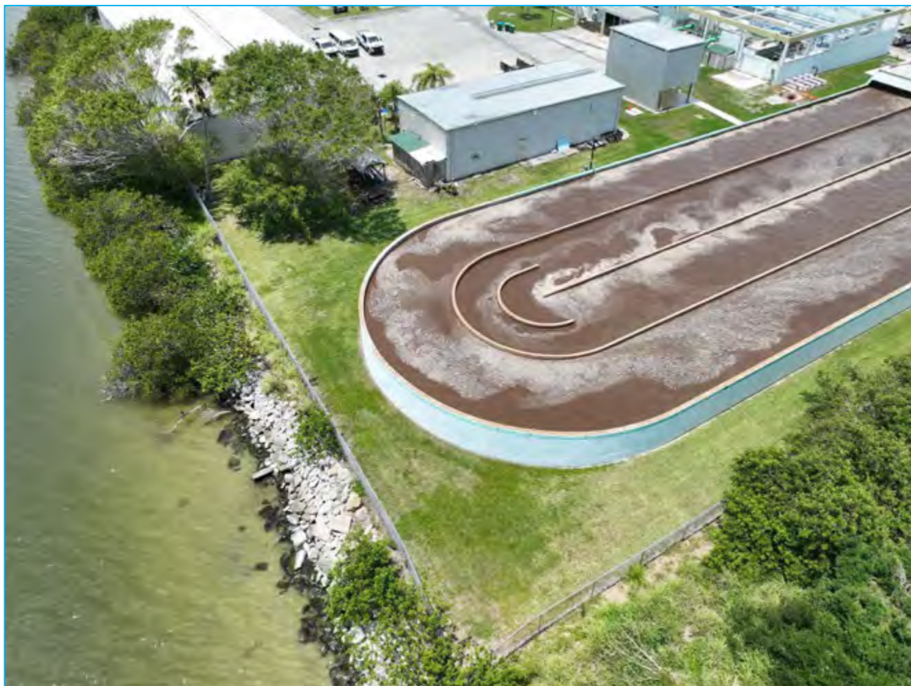
Figure 11. The WRF's Oxidation Ditch is located adjacent to the BRL. Less than 15 feet remain from the southern tip of the Oxidation Ditch to the waters of the lagoon.
