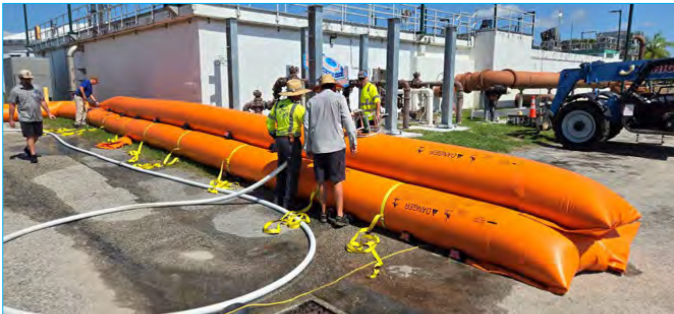
Figure 21. Example of a water inflated temporary dam system.
