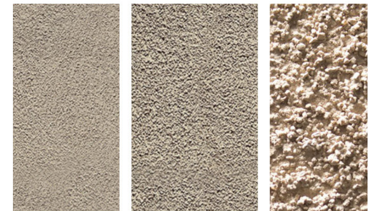
Stucco should have a smooth, not coarse, texture.
