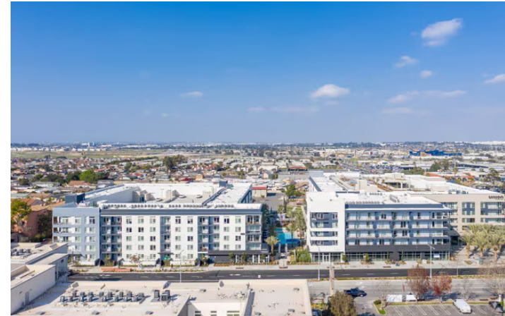
Figure 3 615 E. Carson – Union South Bay
