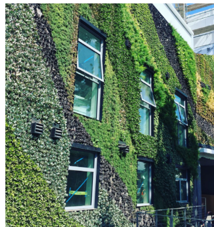
Modular soil cells attached to wall
