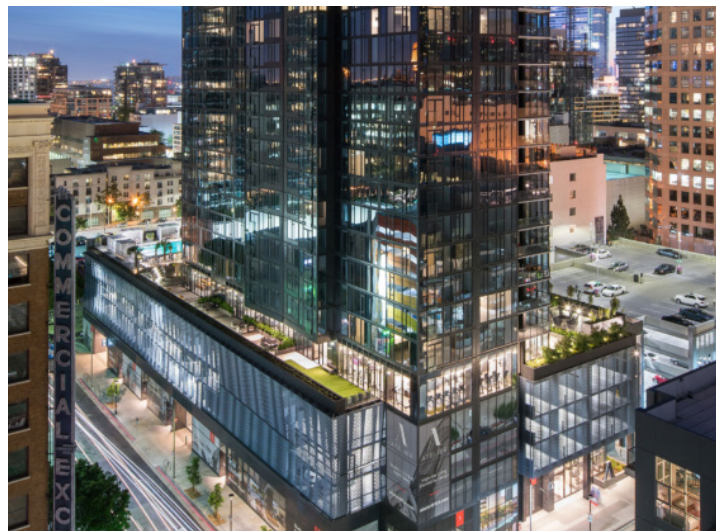
Bridging ground floor activity with upper floor treatment
