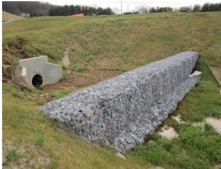
Figure 7.31-2C Forebay with Porous Berm (Gabion Rock)
