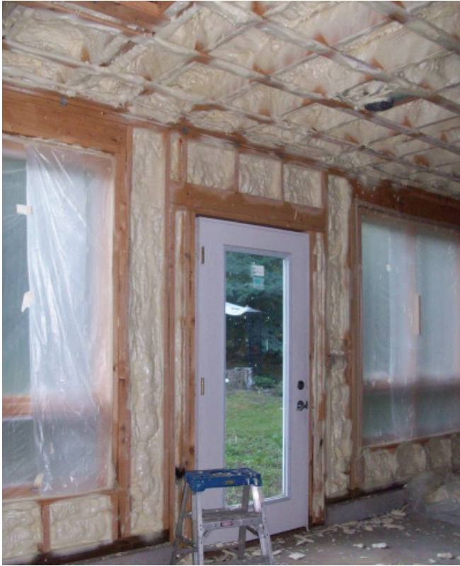
Some building techniques, like spray insulation as compared to blanket insulation, provide better sound attenuation levels. Many of these techniques can also reduce long-term energy costs. Picture courtesy US Department of Energy
