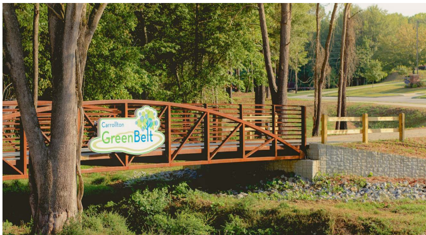
Prefabricated steel bridge allows the trail to cross above existing roads and waterways.
