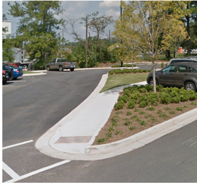
Existing conditions photo of the southern terminus - preferred stop and turn-around location
