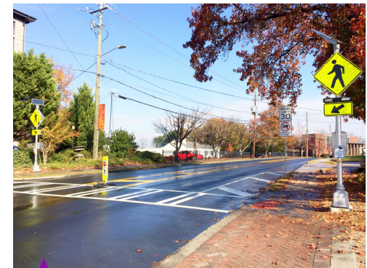
Existing condition photo of the RRFB pedestrian signal at 5424 Peachtree Road
