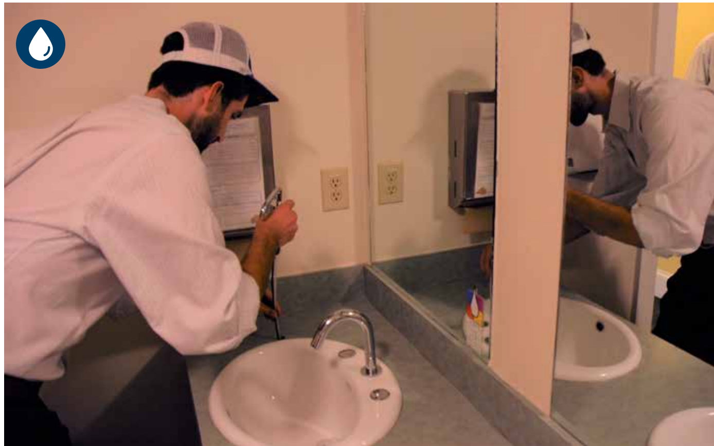
Auditing a sink for potential issues
