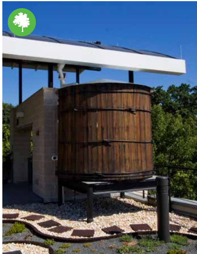
A roof-top cistern
