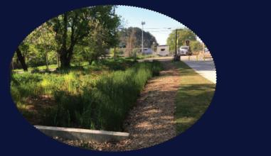
Figure 3.5h – Stormwater swale
