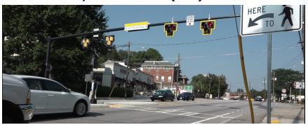
A Pedestrian Hybrid Beacon (PHB) is proposed at Rail-Trail crossings where a conventional traffic signal may not be warranted but traffic volumes, speeds, and crossing distances are unsafe for pedestrians and cyclist to cross unsignalized. PHBs are a candidate crossing signal for roads with:
