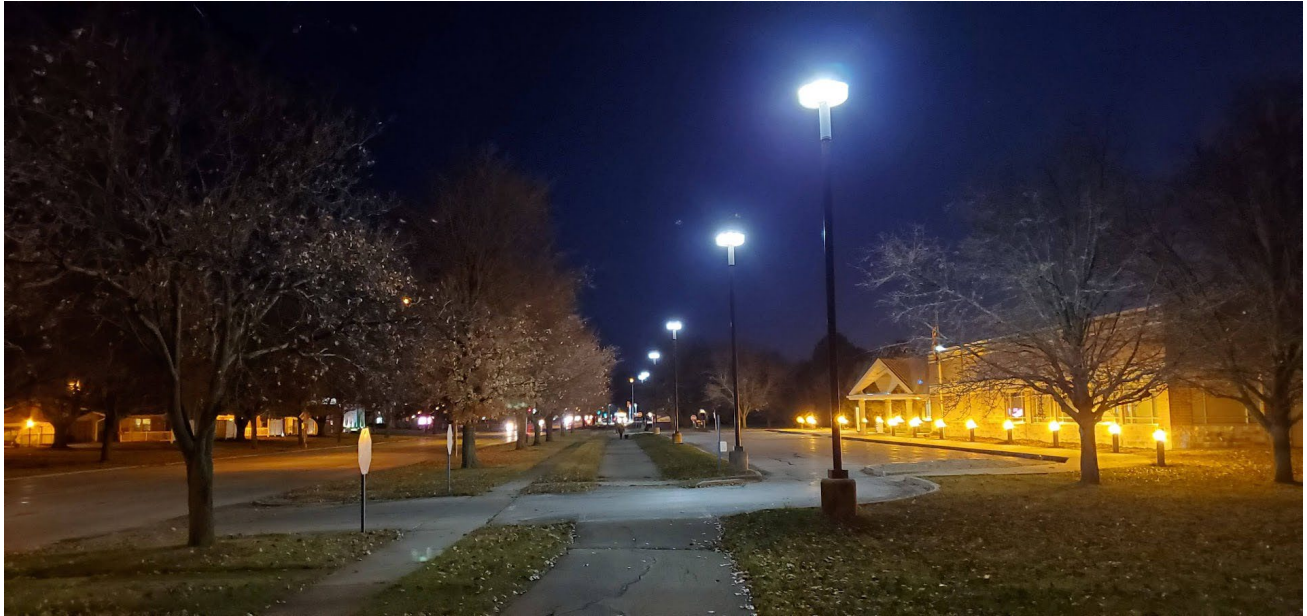
Outdoor lighting at the Rantoul post office
