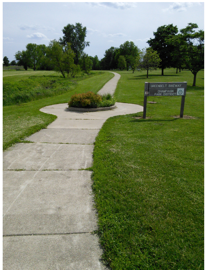
Figure 7-13: Substandard trail width along Greenbelt Bikeway in Heritage Park
