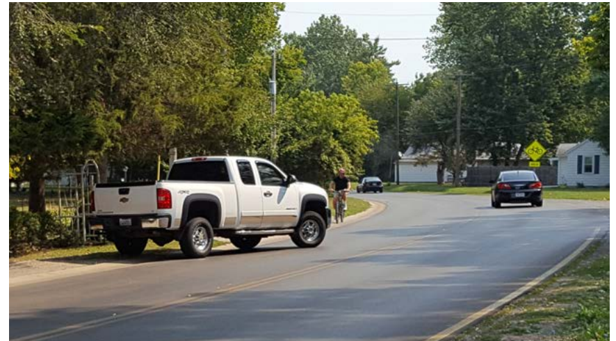
FIGURE 2-19 Lack of separation between bicyclists and vehicles on East Main Street
