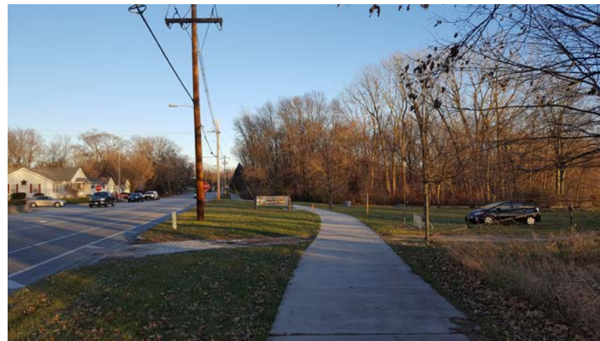
FIGURE 5-2 Main Street Sidepath in Weaver Park
