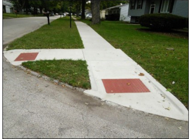
FIGURE 4-1 Sidewalk and Curb Ramps with truncated domes
