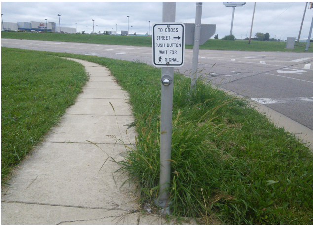
FIGURE 3-30 A low compliance pedestrian push button the southwest corner of Cunningham Avenue and Napleton Way
