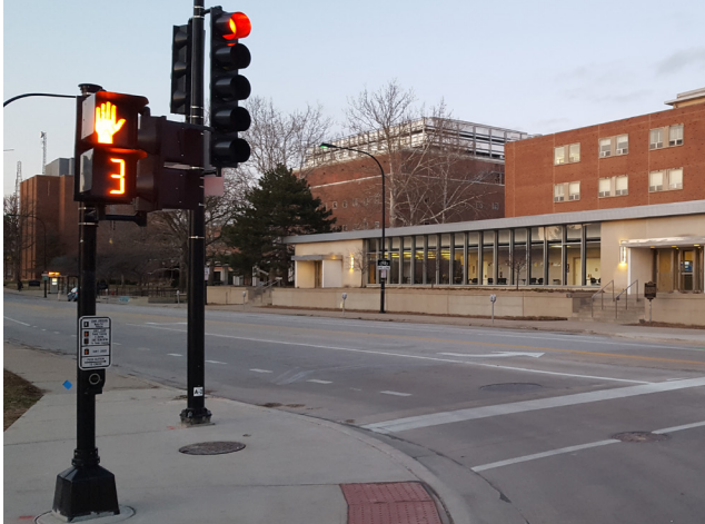
FIGURE 3-29 A high compliance pedestrian signal on the northwest corner of Green Street and Goodwin Avenue
