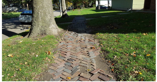
FIGURE 6-11 Brick sidewalk upheaved by tree roots on Elm Street in Historic East Urbana
