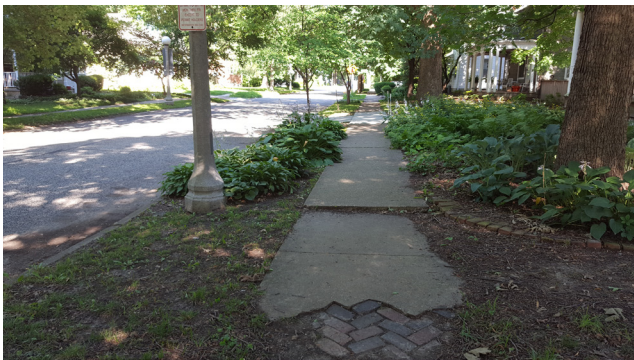
FIGURE 6-1 Uneven sidewalk panels on Oregon Street in West Urbana
