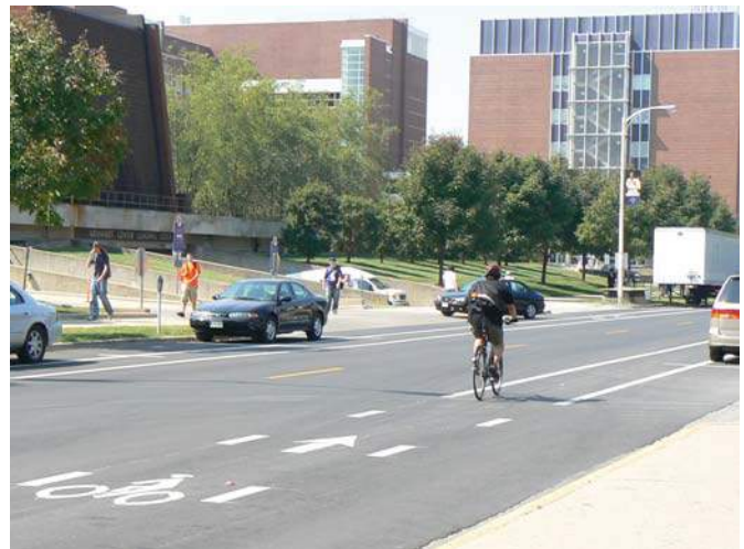
Bikeway: Bike lane on Illinois Street, Urbana
