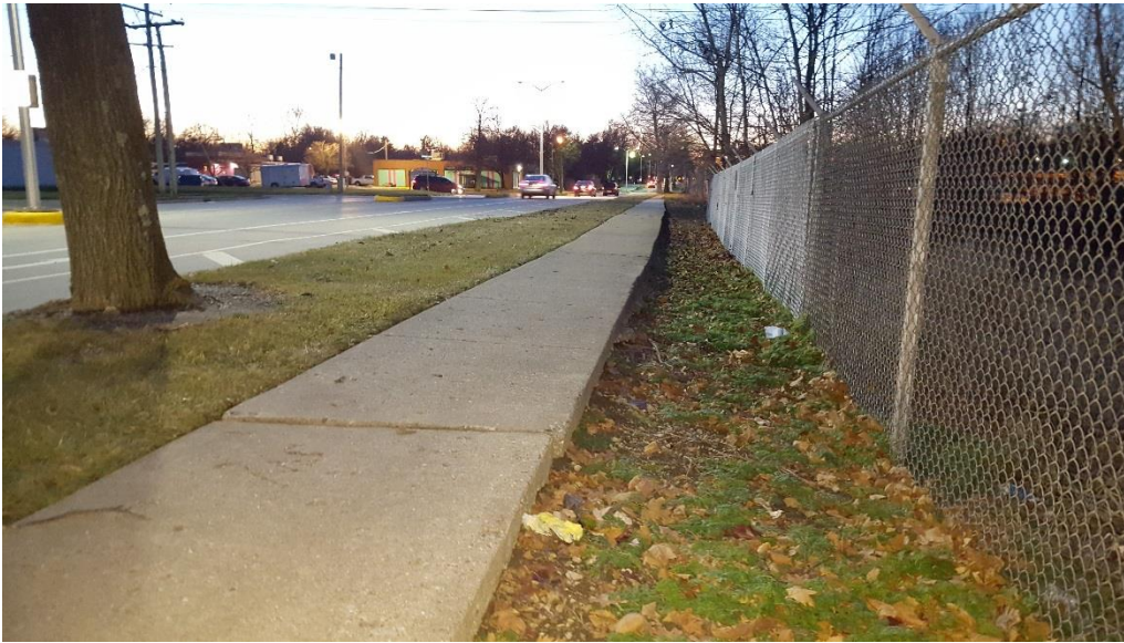
Washington Street north sidewalk westbound between Lierman and Glover Avenues, where several inches separate the top of the sidewalk and the ground to the right.
