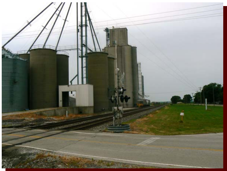
Rail crossing at Milmine
