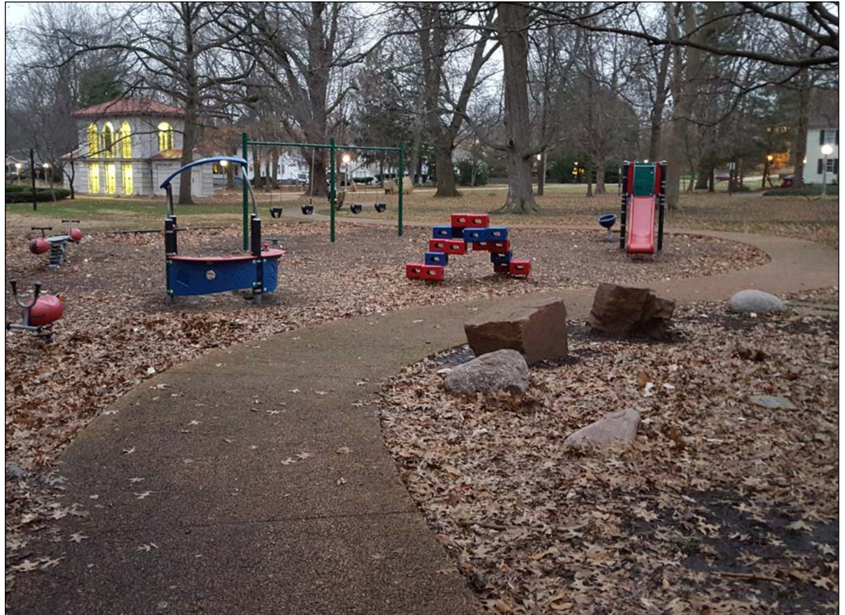
Photo: Permeable sidewalk at Carle Park, Urbana, Illinois, Champaign County Regional Planning Commission
