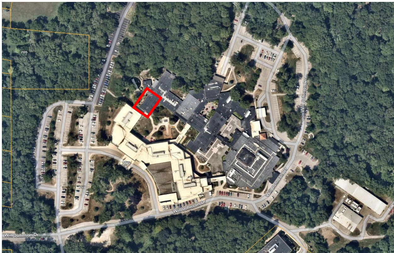
Figure 1. Aerial view of Courtyard West building and surrounding hospital campus
