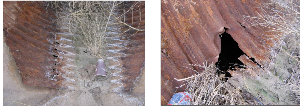
Holes corroded in the culvert pipes under George Hanosh Boulevard
