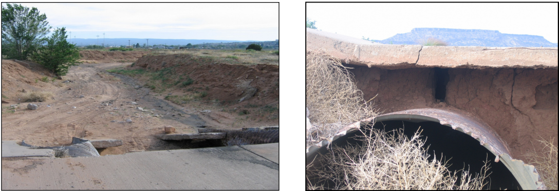
Ends of the existing College Boulevard culverts showing significant deterioration
