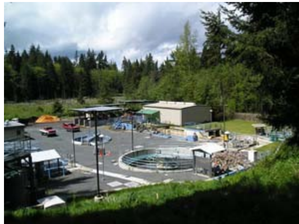
Granite Falls Wastewater Facility
