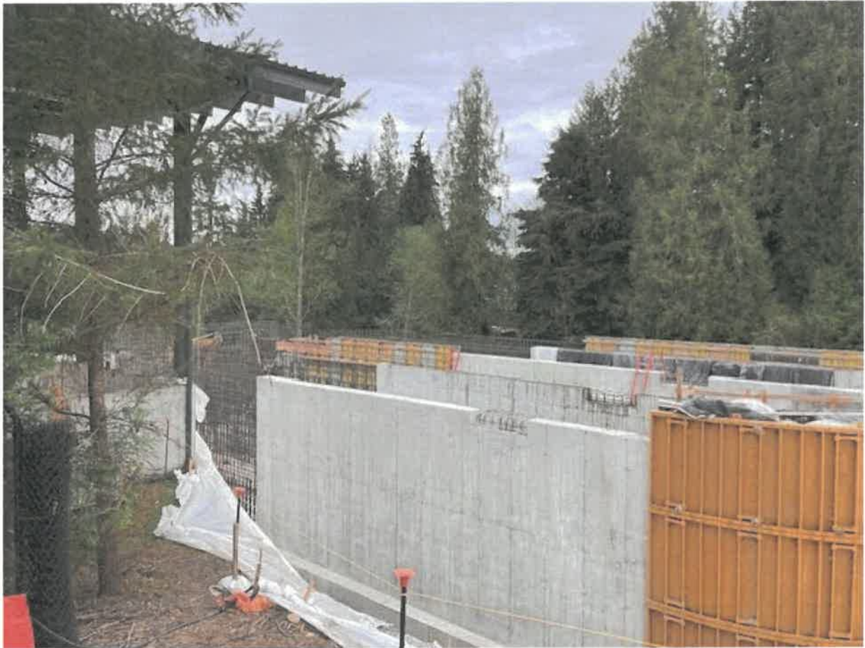
New Oxidation Ditches partially poured:
