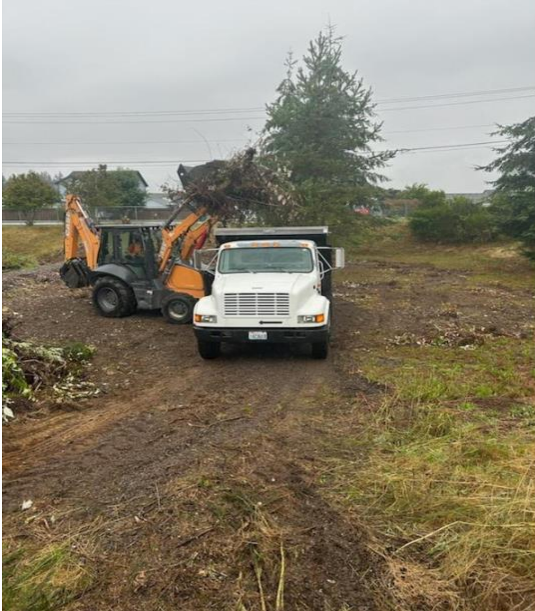
Public Works loading brush at the Pine Lane detention pond.
