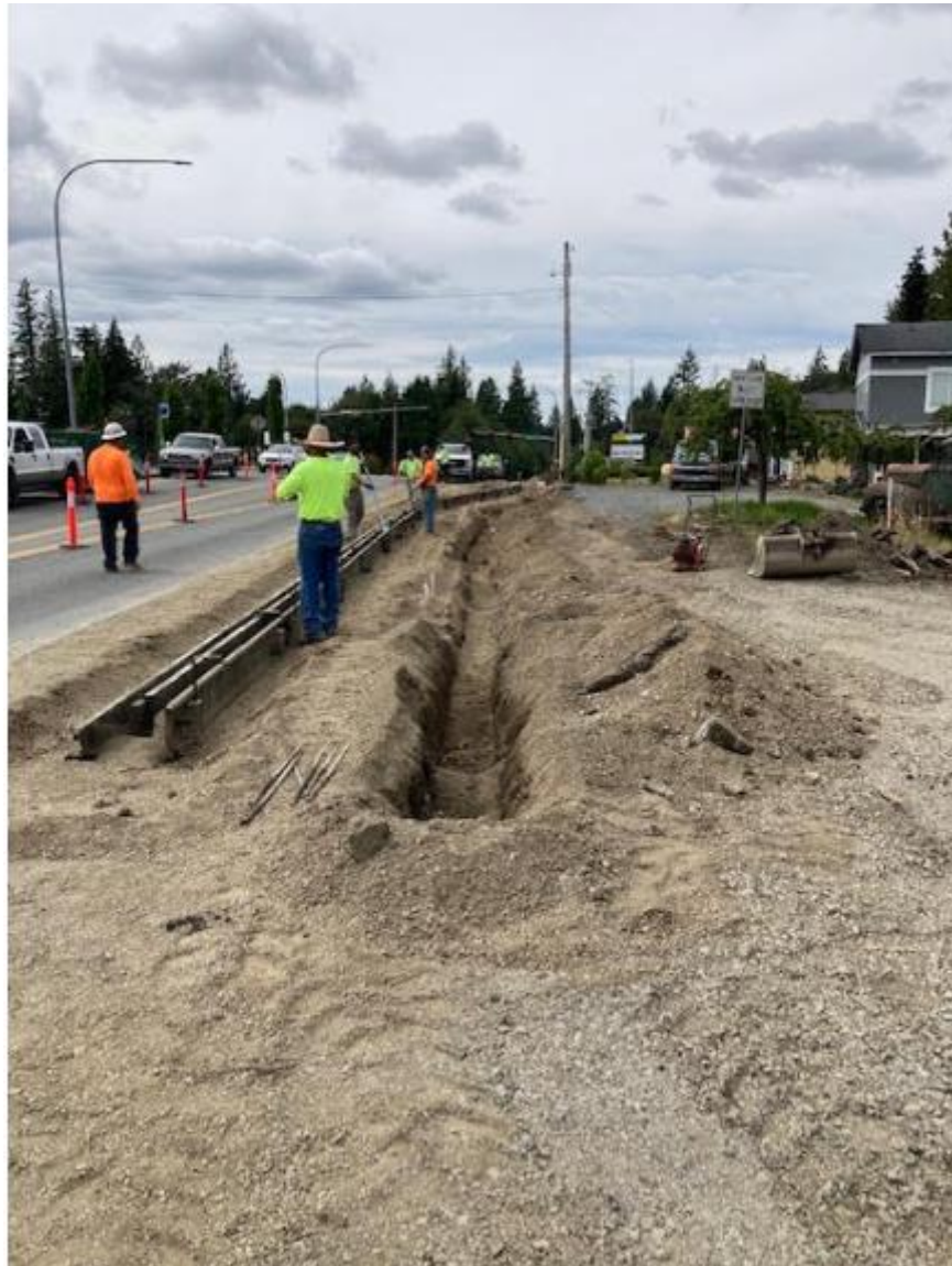
Curb and gutter forms awaiting concrete.
