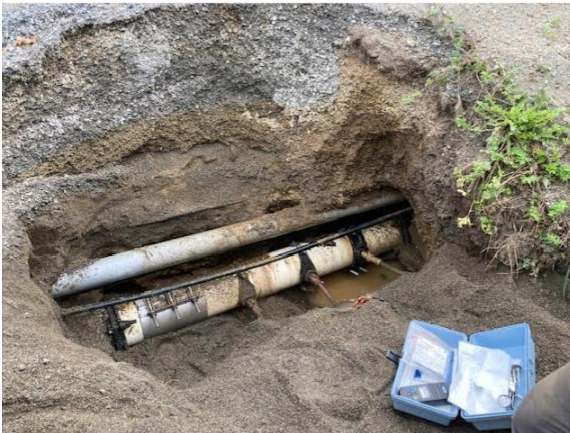
Repair area of the waterline.
