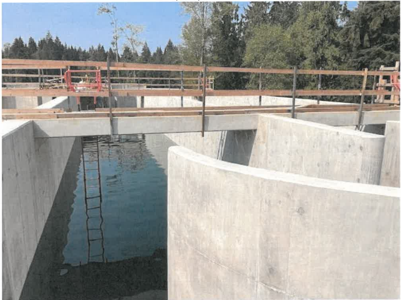
New oxidation ditches partially filled with water for a leak test
