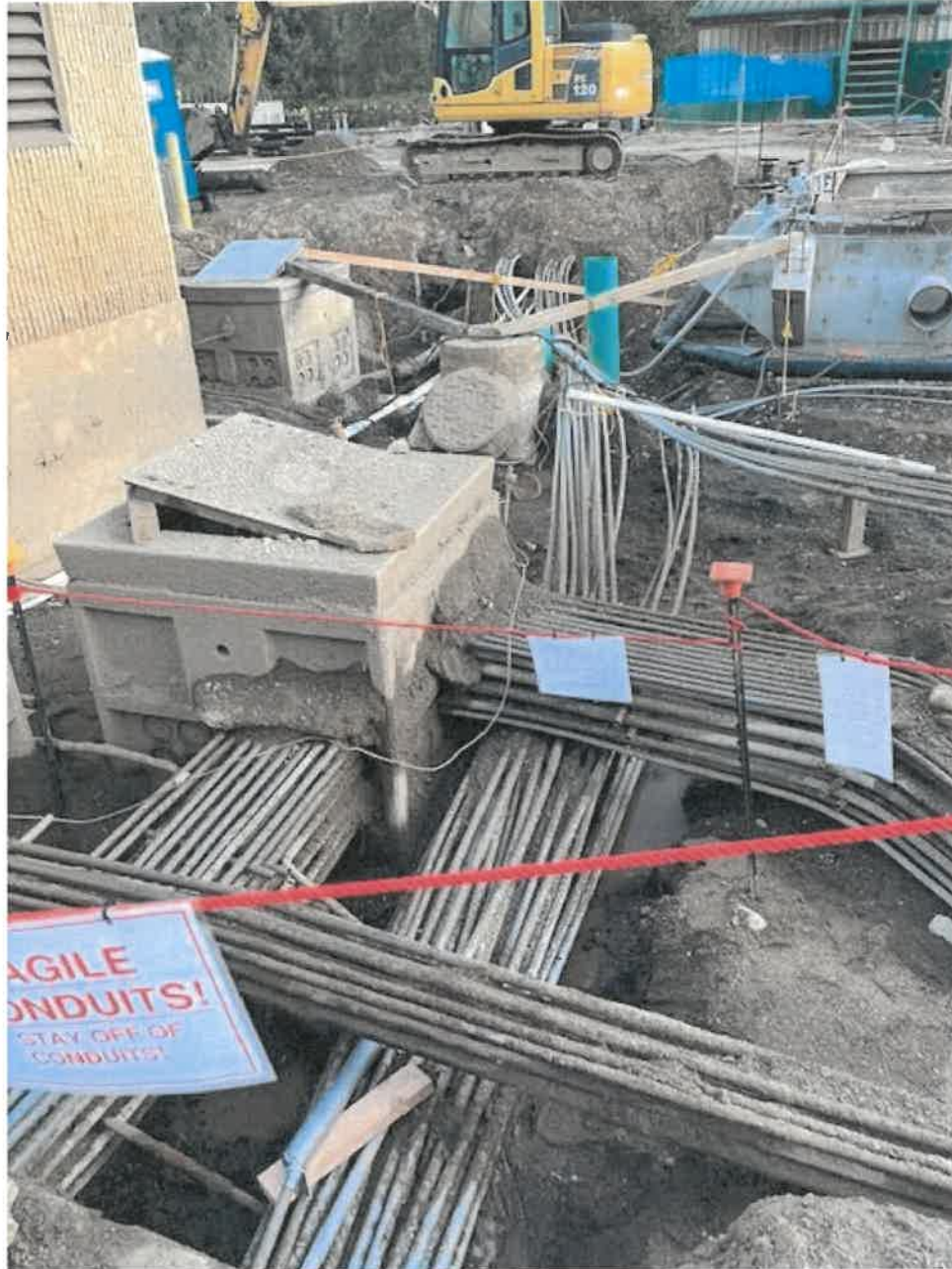
Exposed existing conduit near the op's building
