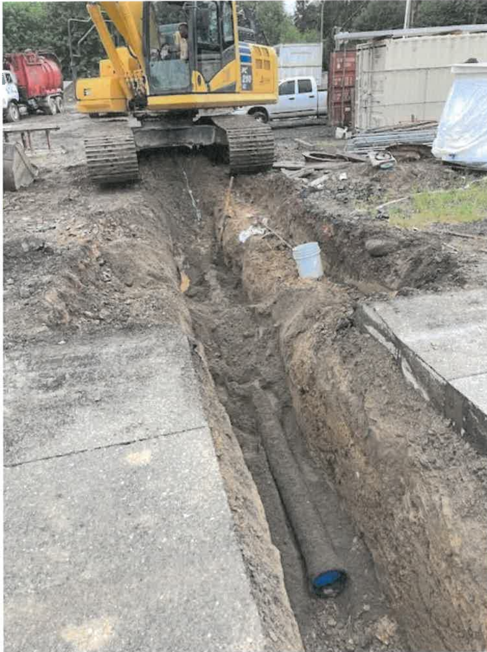
New water line at the N/E corner of the McDaniel's site:
