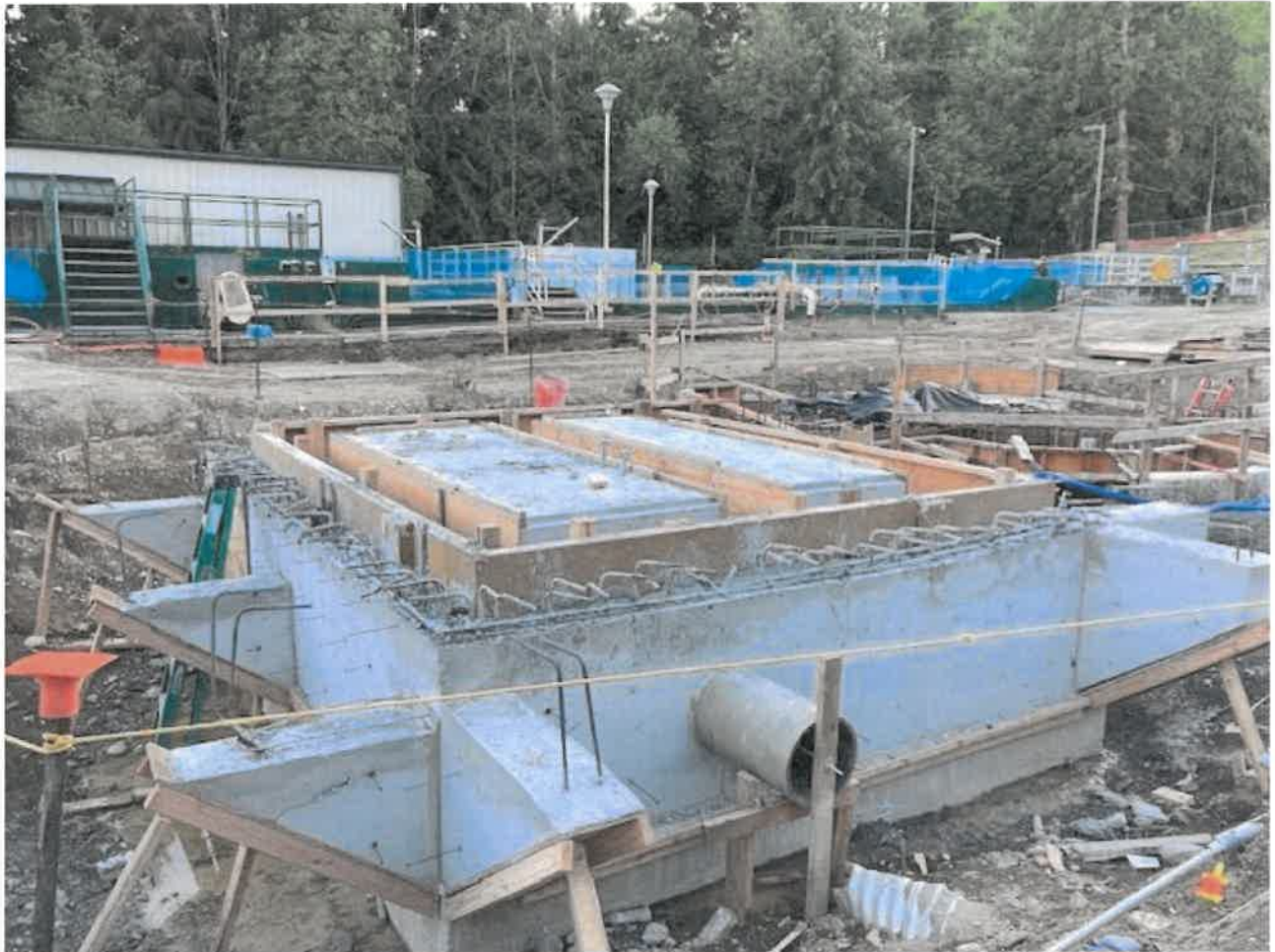
New influent headworks under construction:
