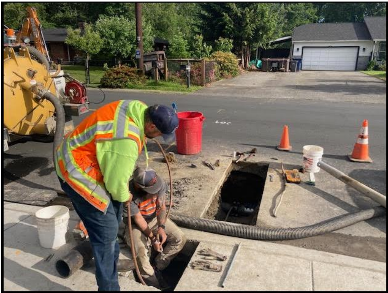
PUBLIC WORKS EMPLOYEES INSTALLING A NEW SERVICE LINE FOLLOWING THE SADDLE REPLACEMENT:
