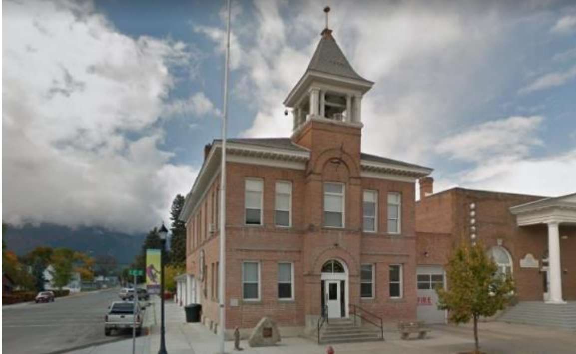
East elevation and main entrance. (City of Hamilton)
