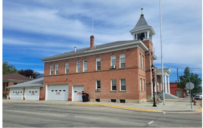
South elevation and garage doors. (A&E Design)
