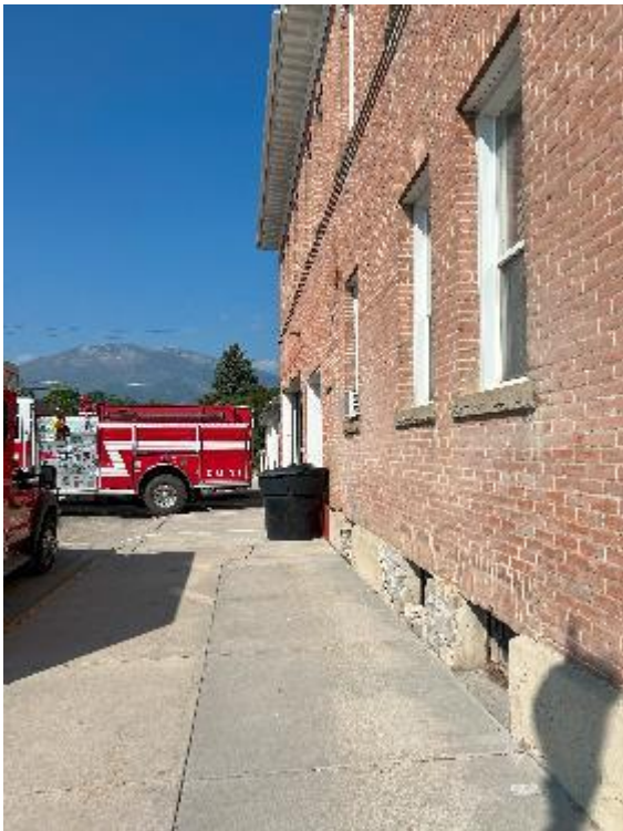
Figure 7 – South façade exterior lighting
