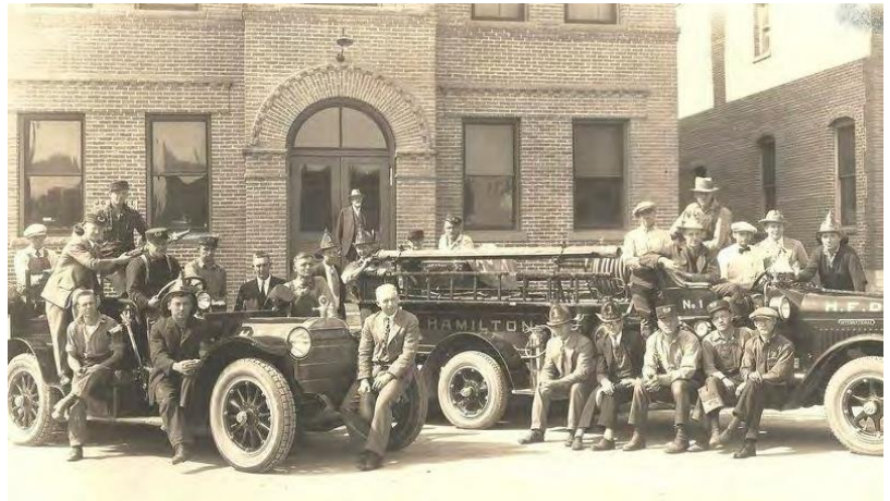
East, main entrance elevation c1930s. (City of Hamilton)
