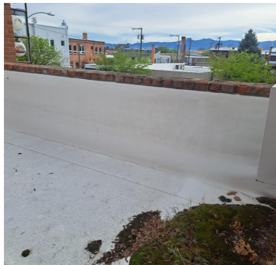
Roof of the north apparatus bay view looking east (A&E Design).
