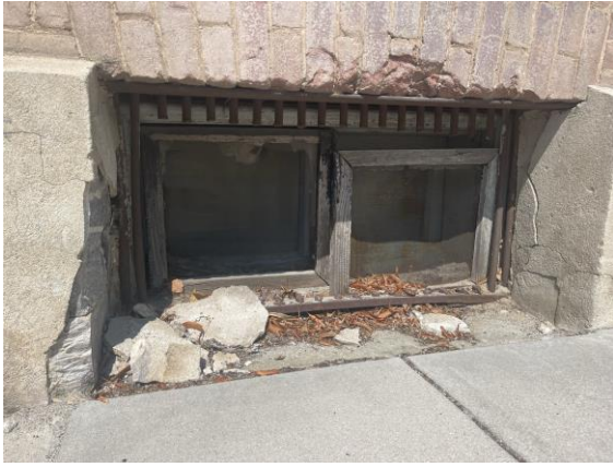
Failed exterior paint finishes, window frame deterioration and damage, and failed concrete parge coating on rusticated cut stone base. (A&E Design)
