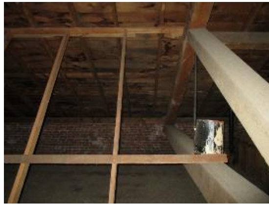
Picture 3: Timber Truss
