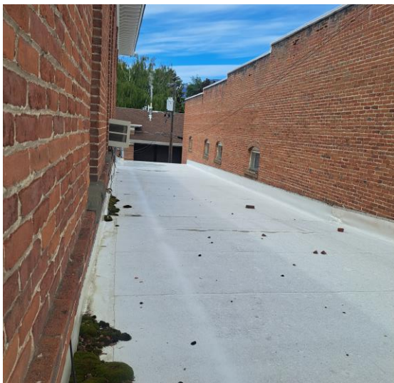
Roof of the north apparatus bay view looking west (A&E Design).
