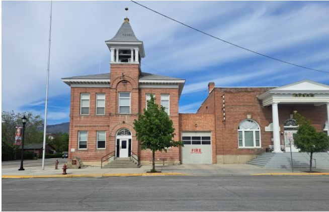
East elevation with garage door infill.
