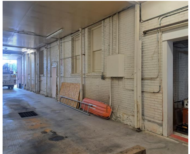
Paint finish on original north elevation windows, frames, and stone base and the non-historic cut opening in masonry wall within the infill that are proposed to be removed with the removal of the north apparatus bay /public way addition. (A&E Design)
