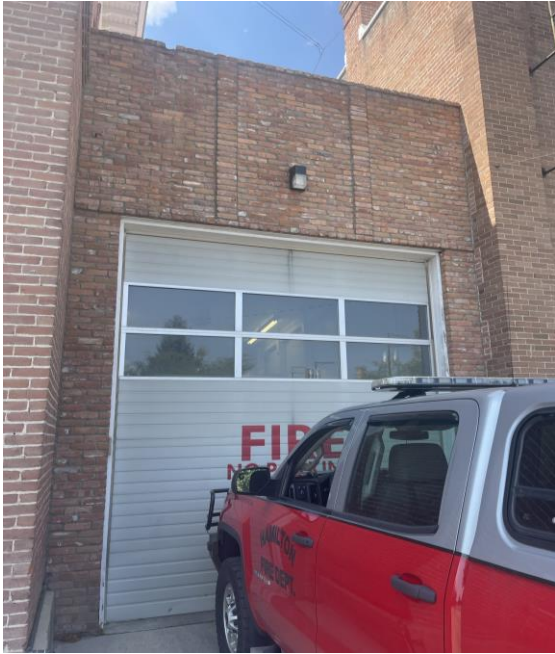
East elevation north apparatus bay addition (to be removed).
