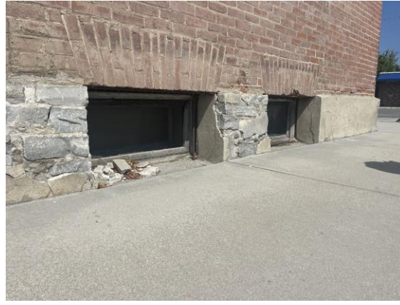
Failed exterior paint finishes, window frame deterioration and damage, and failed concrete parge coating on rusticated cut stone base. (A&E Design)
