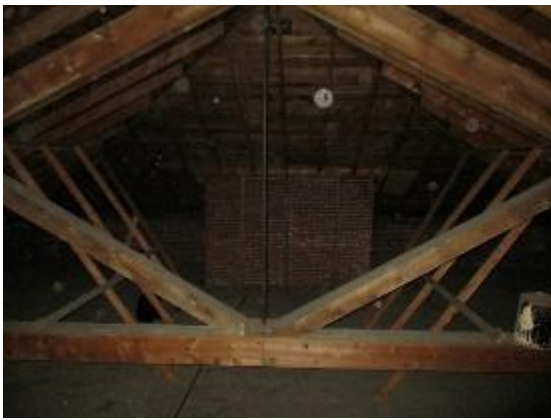
Picture 4: Timber Truss
