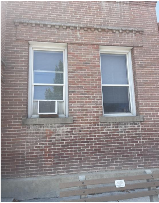
Non-historic window units, metal cladding over exterior brickmold and window frame, and deteriorated exterior paint finishes. (A&E Design)
