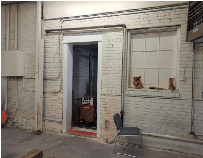
Paint finish on original north elevation windows, frames, and stone base and the non-historic cut opening in masonry wall within the infill that are proposed to be removed with the removal of the north apparatus bay /public way addition. (A&E Design)
