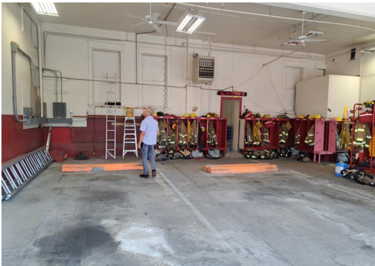
Historic Town Hall, Garage Bay, refer to electrical and mechanical equipment.
