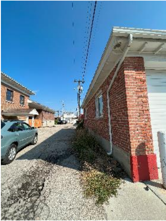
Figure 1 – NWE’s overhead distribution
