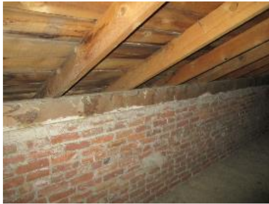
Picture 2: Roof rafters on timber rim
