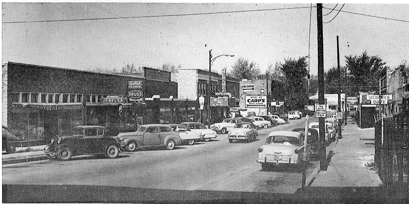
Looking North - North Clark Street - Today
