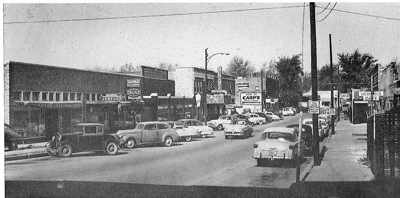
Looking North - North Clark Street - Today
