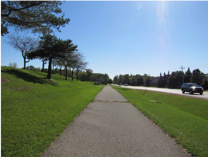
Separated 8-Foot Pathway: This facility will serve riders at all levels of traffic stress tolerance.
