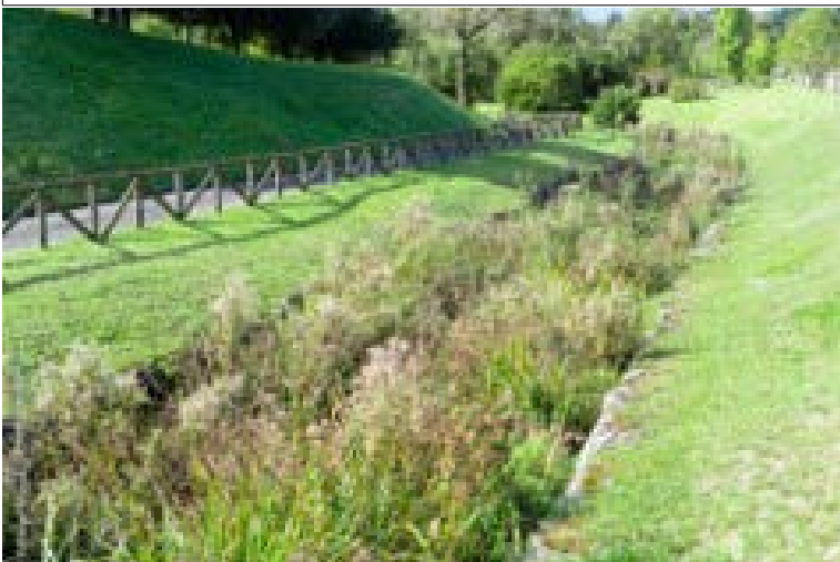
Bioswales such as the one above can help manage stormwater and runoff and are planned to be installed throughout the Eastern Market District in Detroit.
