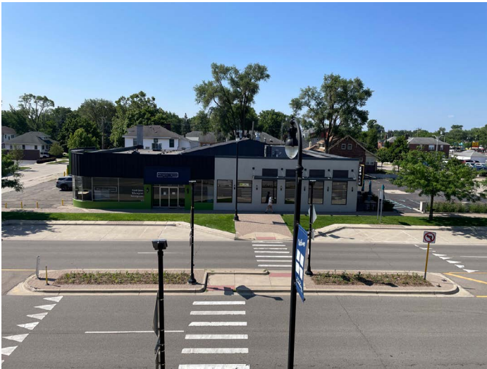
Pedestrian Island with Signal: Clawson has three such signals in its Downtown.
