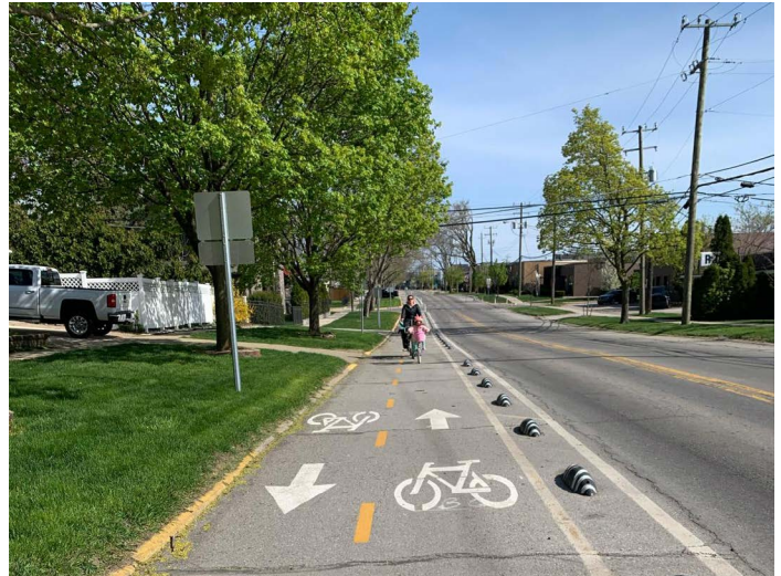
Protected Bike Lane: This facility will serve all but the most cautious riders.
